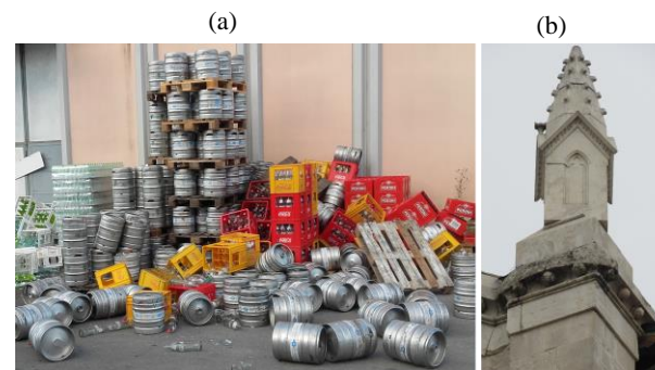
Figure 1: Post-earthquake damage (after the 24/08/16 Amatrice earthquake, Italy) of critical unanchored elements: (a) overturning of beverage stocks; and (b) rigid dislocation of the pinnacle of the San Benedetto Basilica .
