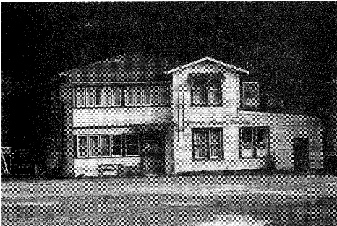
Figure 4(b): A typical pre-1968 two storey hotel of house style construction, with a corrugated iron roof, weatherboard wall cladding and piled foundation.
