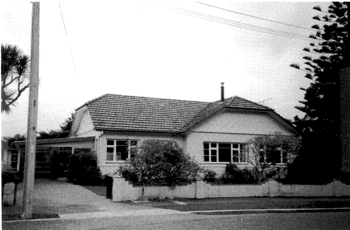
Figure 3(b): A pre-1968 one storey West Coast house with tiled roof, stucco veneer walls and concrete strip foundations.
