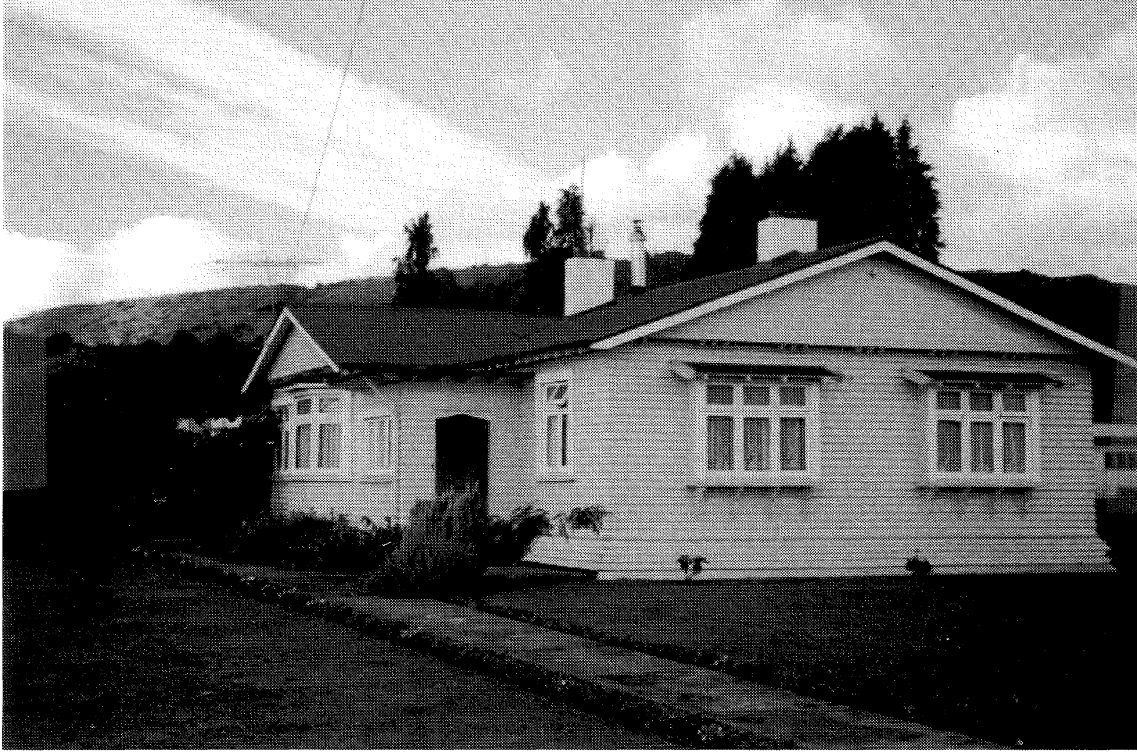
Figure 3(a): The most common type of pre-1968 West Coast house, one storey with a corrugated iron roof weatherboard wall cladding and piled foundations.
