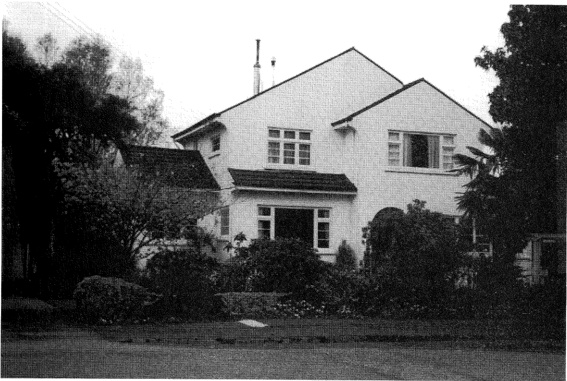
Figure 4(a): A pre-1968 two storey West Coast house with a tiled roof, stucco veneer walls and concrete strip foundation.
