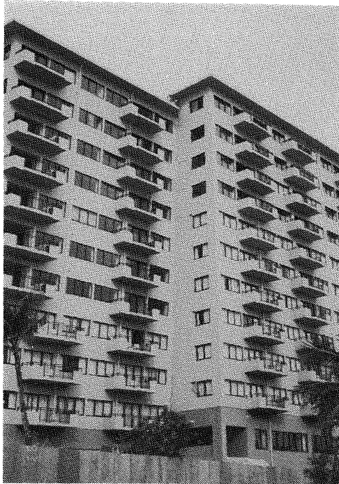
Figure 17 Damage to west wing, Royal Palm Hotel
