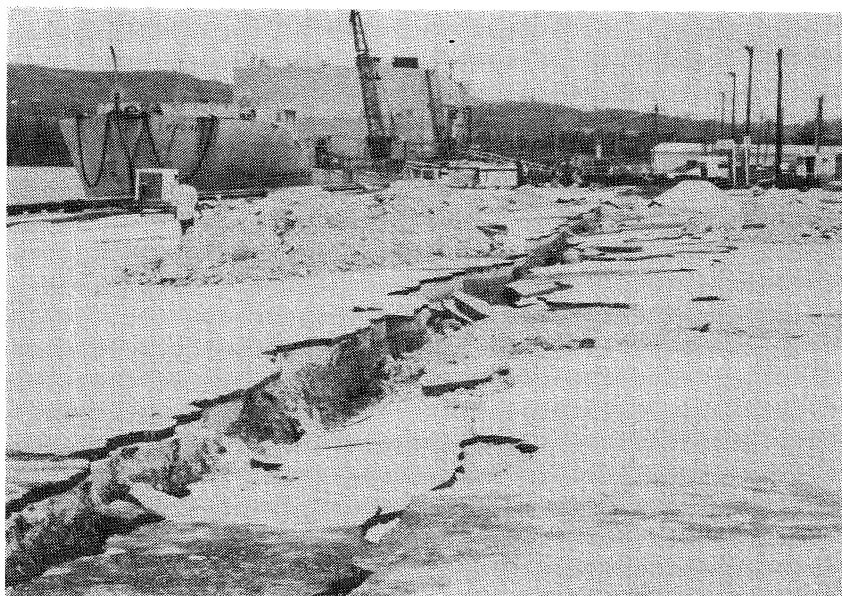
Figure 3 Lateral spreading of US Coastguard port facilities
