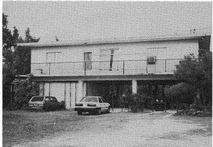
Figure 10 House on free-standing columns
