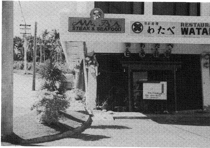
Figure 12 Front of Grand Hotel showing soft storey effects
