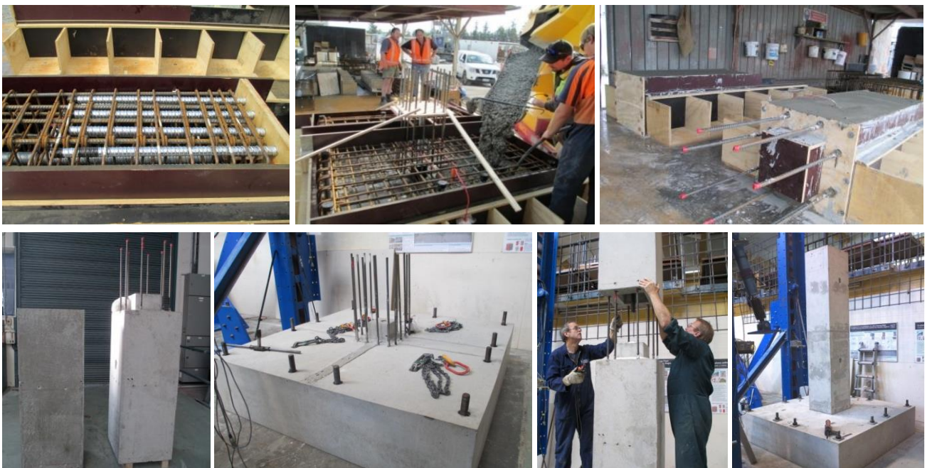
Figure 8. Construction and assembly of HDS1 and HDS2.
