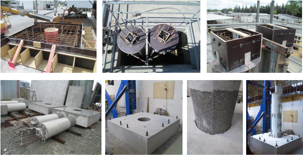
Figure 16. Construction and assembly of HDC1 and HDC2.
