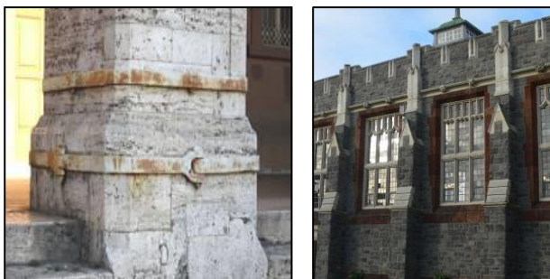
a) Addition of column confinement b) Presence of buttresses
