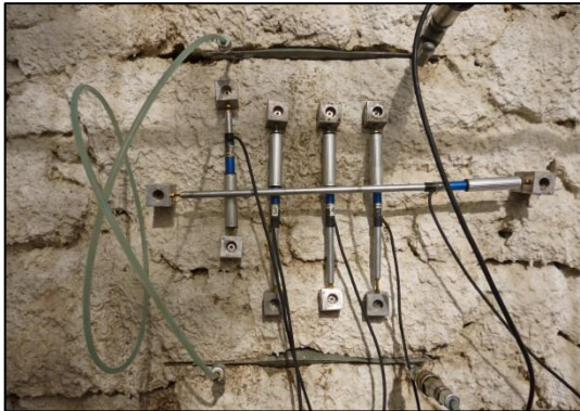
Figure 5: Execution of double flat-jack test [www.expin.it].
