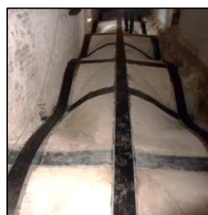
a) Application of FRP on masonry vaults
