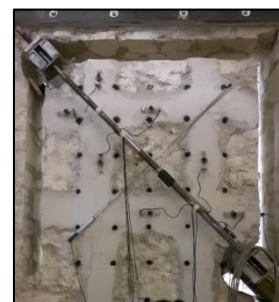
b) Application of TRM on masonry wall
