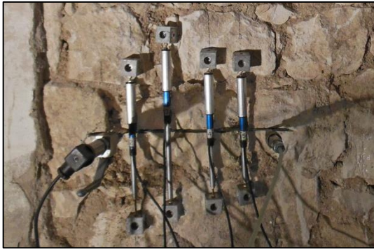
Figure 4: Execution of single flat-jack test [www.expin.it]
