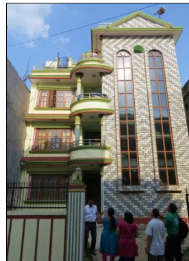
(d) Building clad with tiles and plaster
