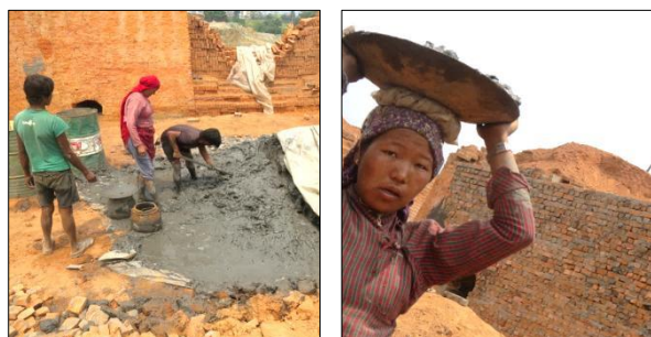
(a) Mud mortar mixing onsite
