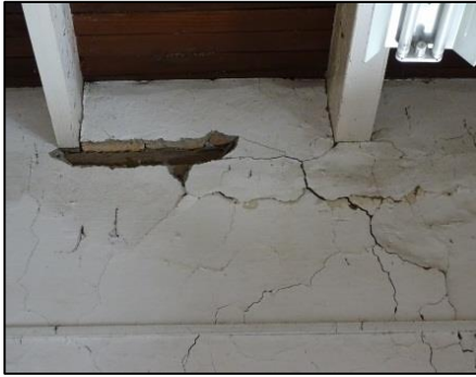
(a) Pull out of the timber joints supporting floor diaphragm
