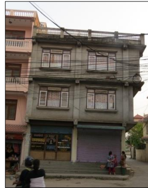
(a) Cantilever/overhanging floor levels resulting in severe elevation irregularity
