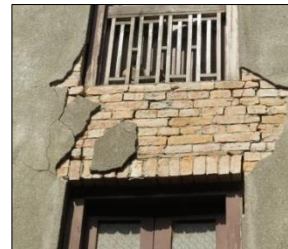
(a) Flexural cracking
