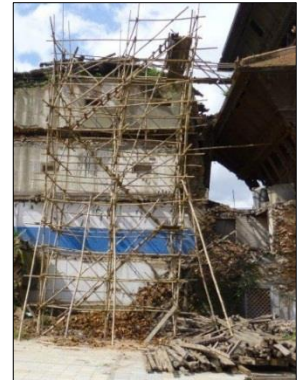
(b) Example of shoring using bamboo members
