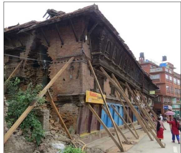
(c) Example of shoring using timber members
