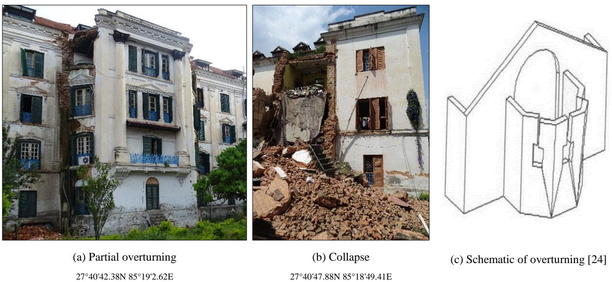
Figure 22: Overturning of the building plan protrusions.
