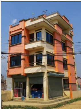
(c) Building finished with rendered plaster and paint
