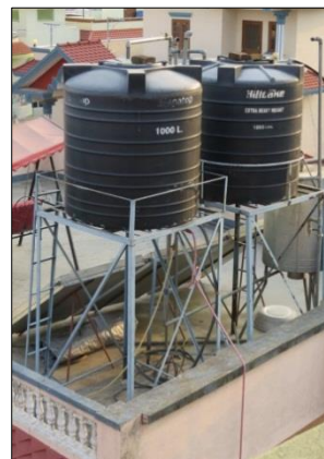
(c) Steel braced frame support frame
