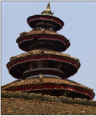
(b) Leaning of top portion of a Pagoda type temple
