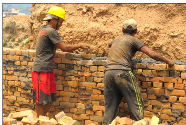
(c) Masonry construction, using English bond pattern and fired clay bricks
