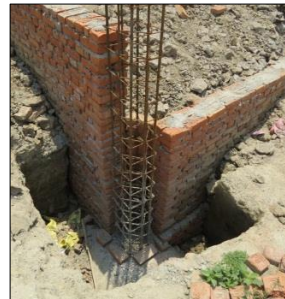
(a) Foundation pit with URM walls and RC column
