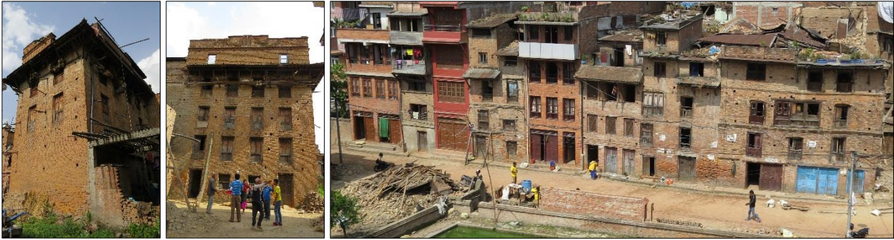
(a) Examples of standalone and row loadbearing URM buildings with mud mortar in poorer residential areas
