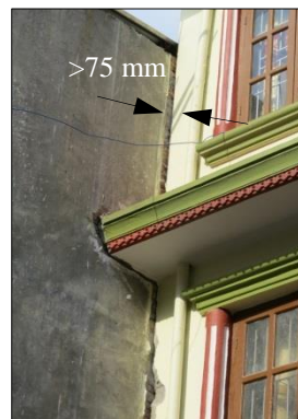
(a) Differential movement due to foundation rotation
