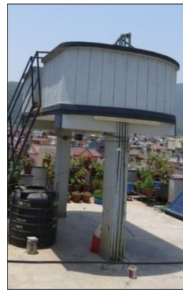
(a) Cantilevered RC support platform
