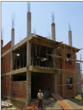
(a) Building during construction
