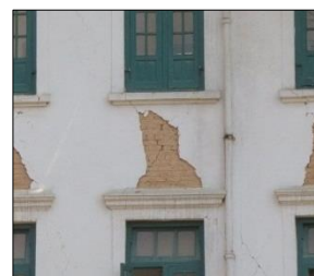
(b) Diagonal cracking
