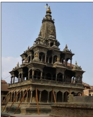
(a) Minor damage in masonry temple
