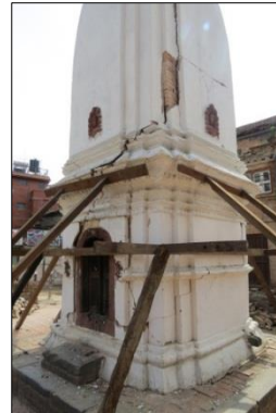
(a) Shoring of a cultural heritage monument
