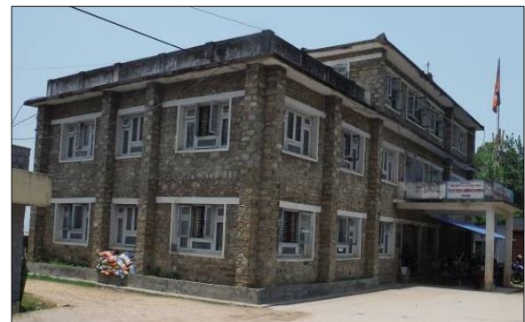
Figure 12: Unreinforced stone masonry building with cement mortar and RC floor and roof diaphragms (minor to no damage observed).
