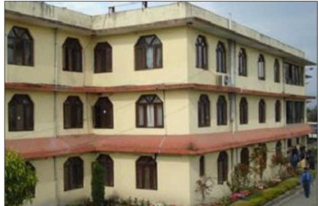
(c) Example of mid-range URM buildings with cement mortar and RC floor and roof diaphragms
