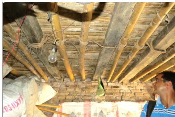
(a) Bamboo floor diaphragms with a heavyweight mud topping (typical domestic URM construction)
