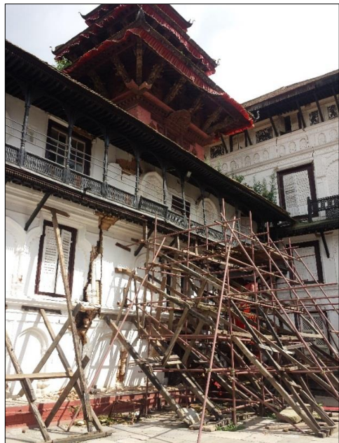
(e) An example of shoring using timber and steel members
