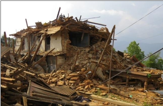
(b) Collapse due to poor quality of the masonry (Chautara)
