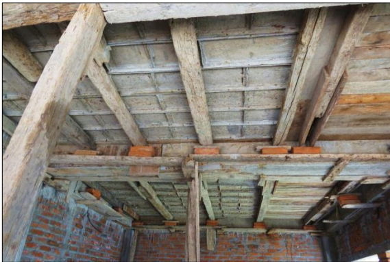
(e) Typical diaphragm used in confined masonry buildings (showing type of formwork used)
