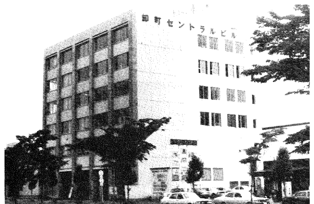
NO DAMAGE TO BUILDING OPPOSITE
