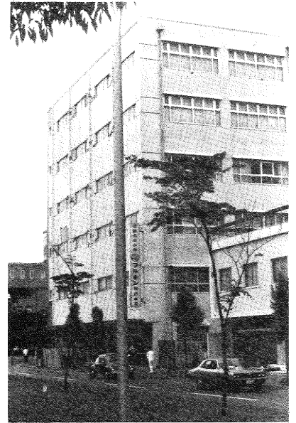
FRONT AND SOUTH SIDE
