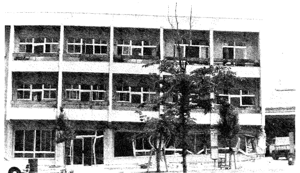
VIEW OF SOUTH WALL
