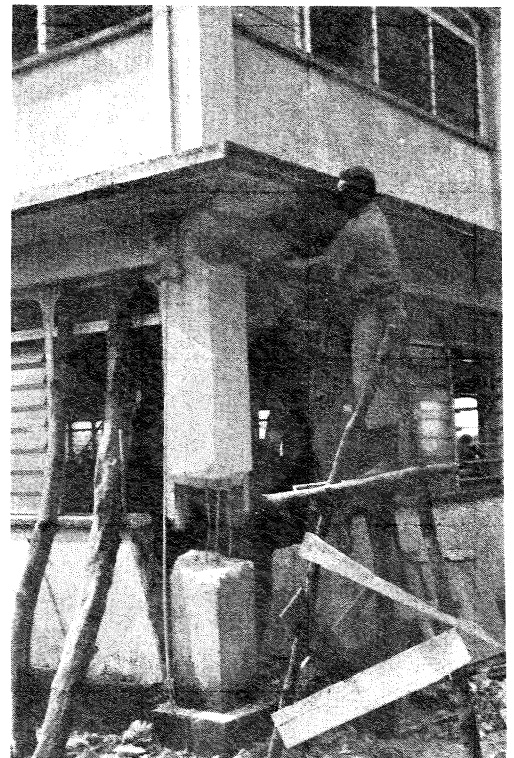
FIGURE 12: CORNER COLUMN UNDER REPAIR - TAILULU COLLEGE
