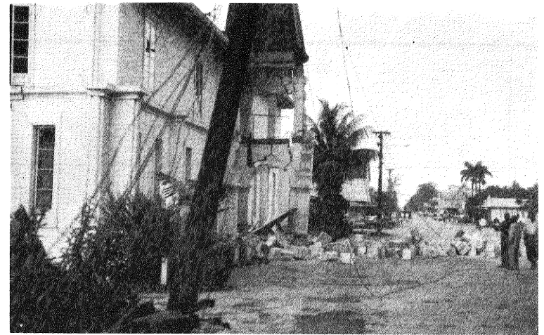
FIGURE 3: PRIME MINISTER'S BUILDING, NUKU'ALOFA. NOTE POWER LINES.
