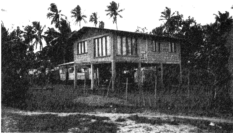
FIGURE 2: HOUSE ON LONG PILES
