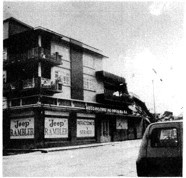
FIGURE 7: COLLAPSE OF THE "PACKARD" APARTMENT BUILDING, ORIZABA.
