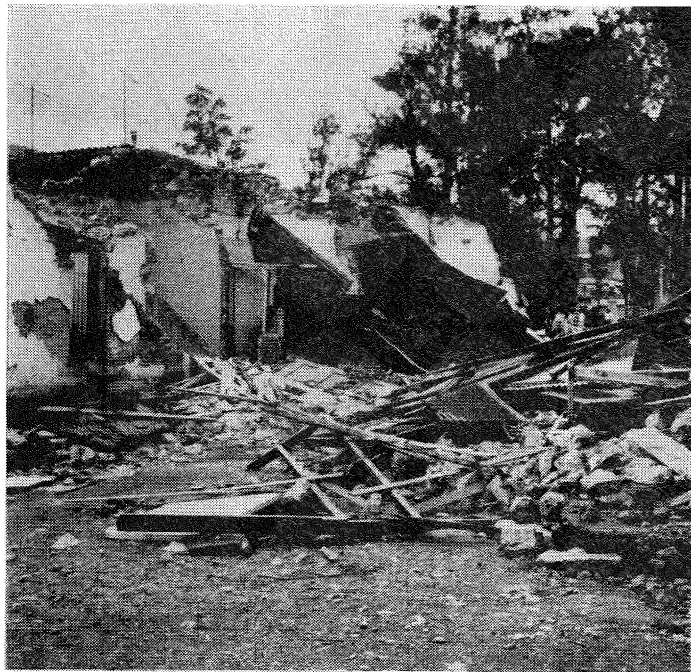
FIGURE 3: COLLAPSED HOUSES, RIO BLANCO.
