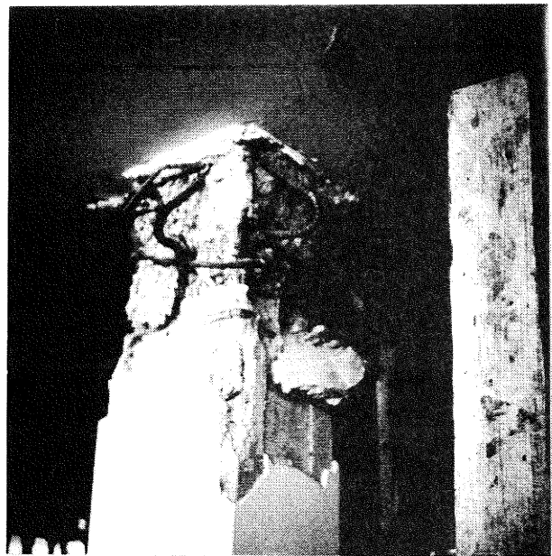
FIGURE 17: AXIAL COMPRESSION FAILURE OF A THIRD-FLOOR COLUMN, BUSINESS HOUSE, CORDOBA.
