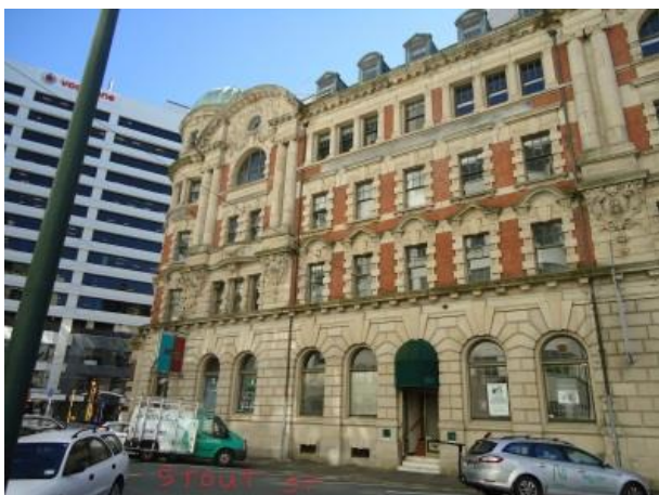
Figure 21: Old Public Trust building in Wellington.
