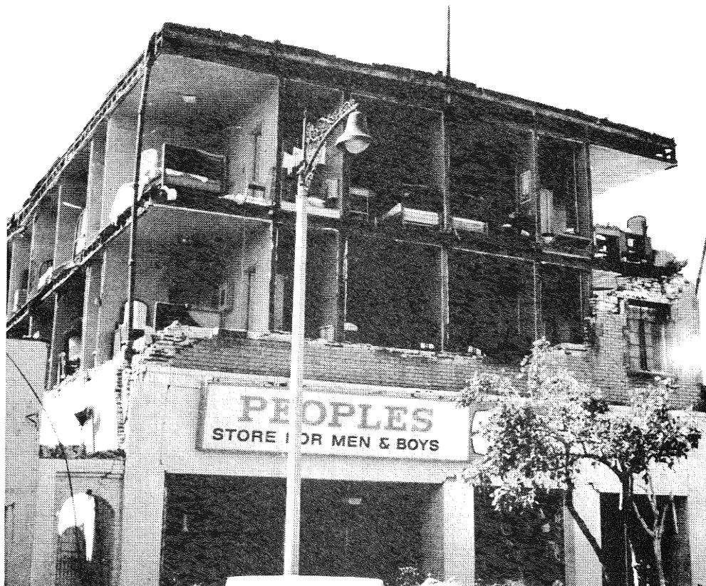
Fig 10. Mission Hotel, San Fernando Mall. Masonry walls
