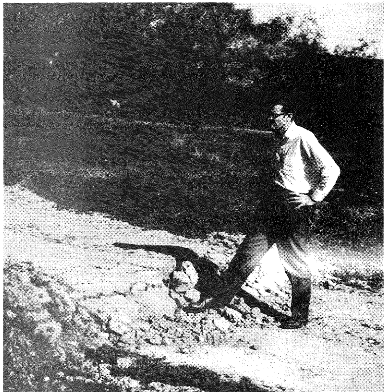
Fig 6. Thrust scarp in fields above end of Pierce Street.
