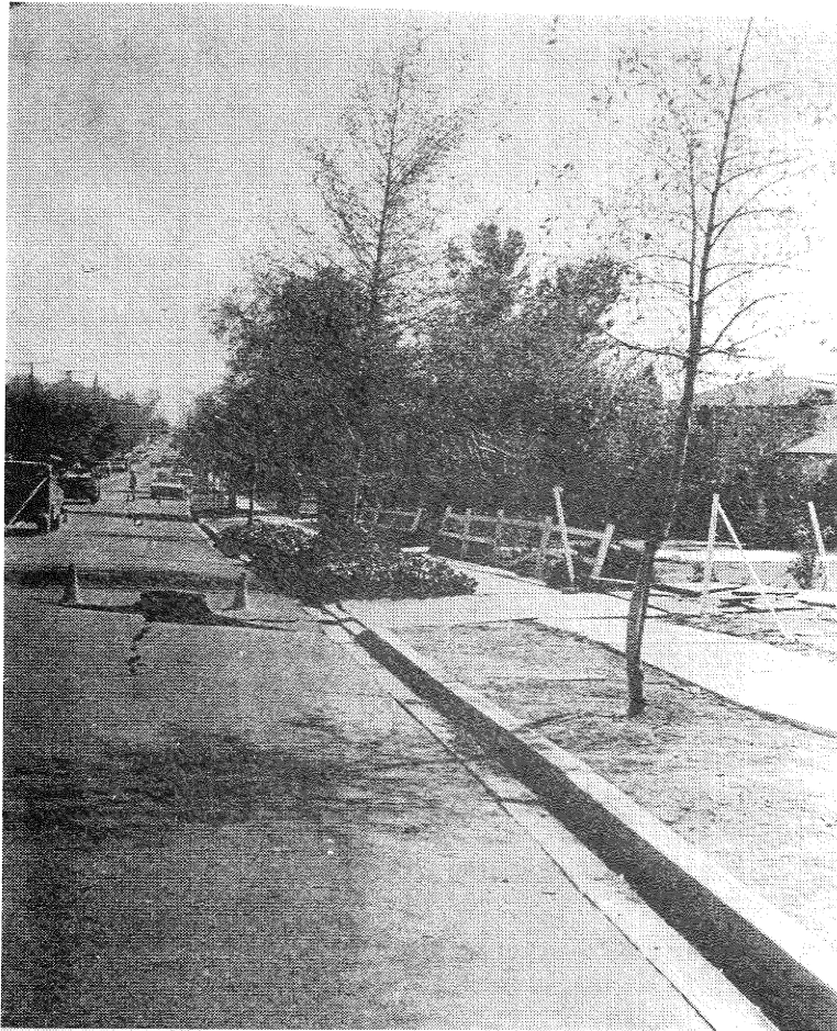
Fig 3. Offset curb looking SE along Eighth Street. Camera is on line of curb in distant part of street.
