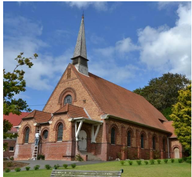
(a) St. Paul's church (1916), Auckland - Clay brick
