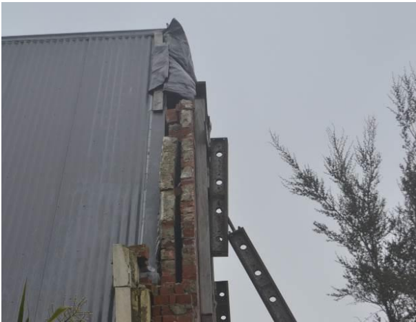
(a) St Joseph's Church (1921), Christchurch – Clay-brick cavity wall
