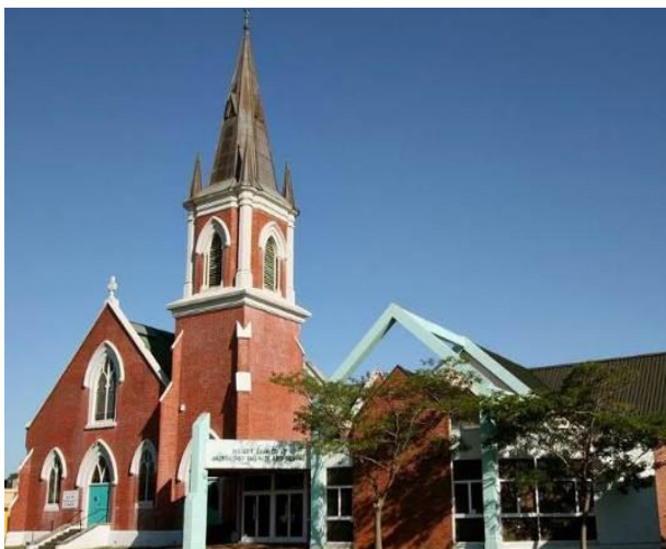
(b) Wesley Broadway Methodist Church (1911), Palmerston North - Presence of adjacent buildings and raised element
