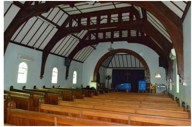
(e) St Andrew's Church (1914), Auckland - Roof partially hidden by ceiling
