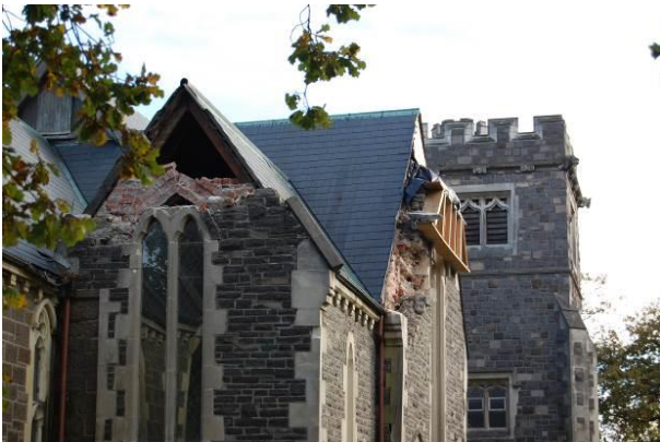
(c) St Peter's Church (1875), Christchurch (Photo courtesy of Joao Leite) - Two-layer wall
