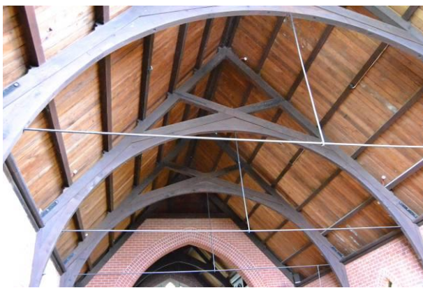
(a) St Luke's (1908), Wellington - Tie rods in the roof
