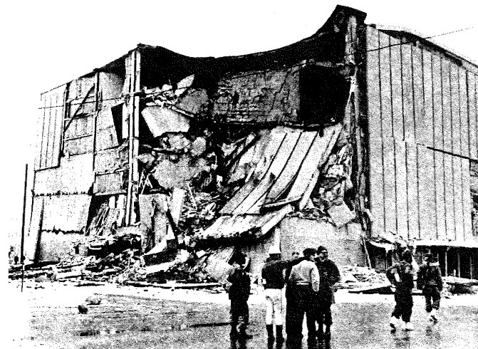
Northeast corner of Penney Building.
