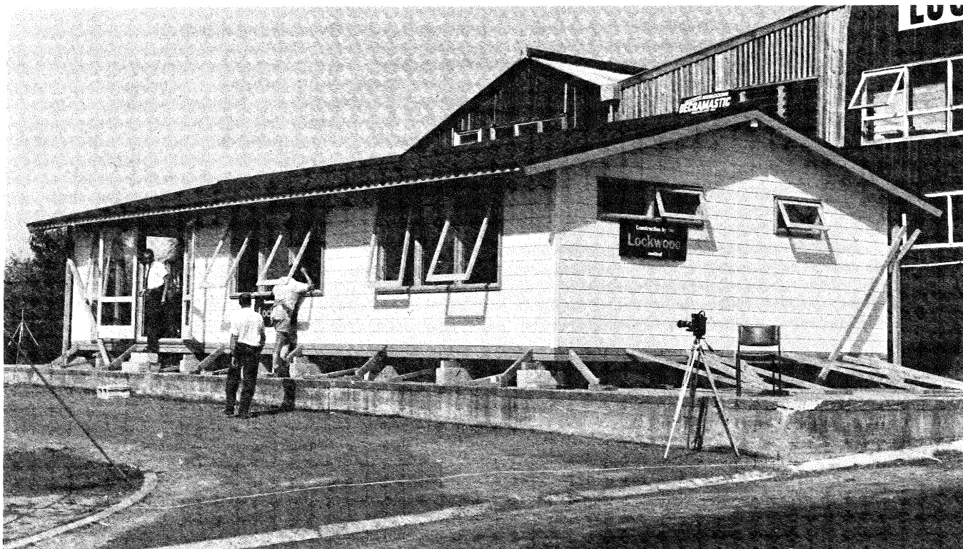
Fig. 4. View of house supported by concrete blocks upon a concrete slab.
