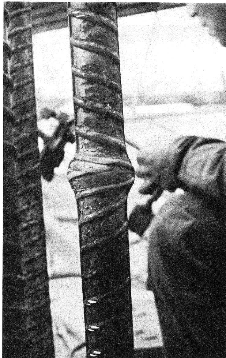
Fig. 6. The completed weld.
