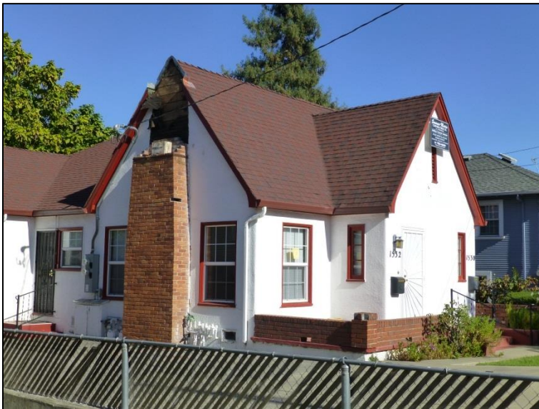
(a) Chimney damage in Napa
