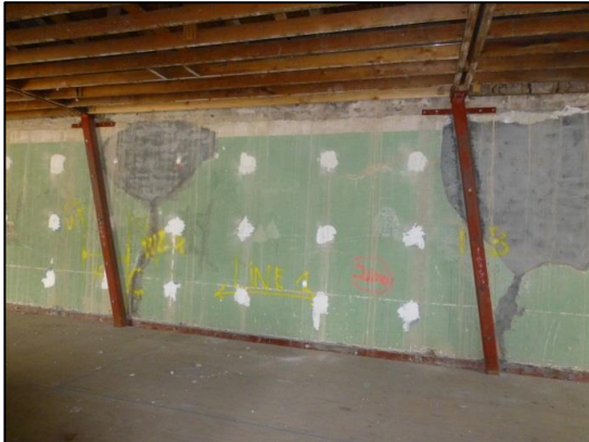
(a) Lay-out of through-wall anchors
