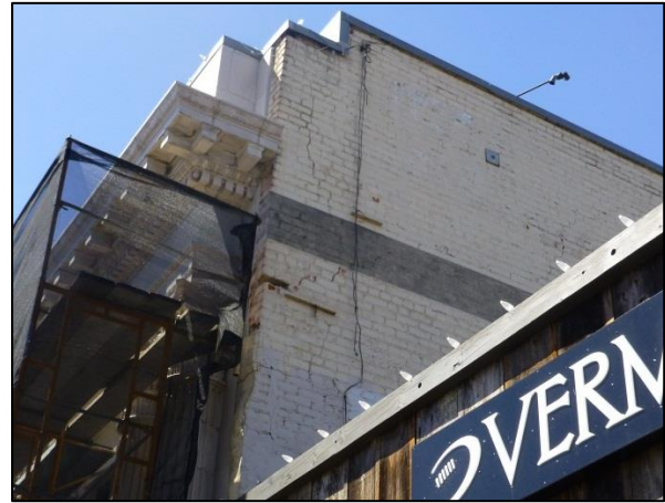
(b) Impending end-wall separation
