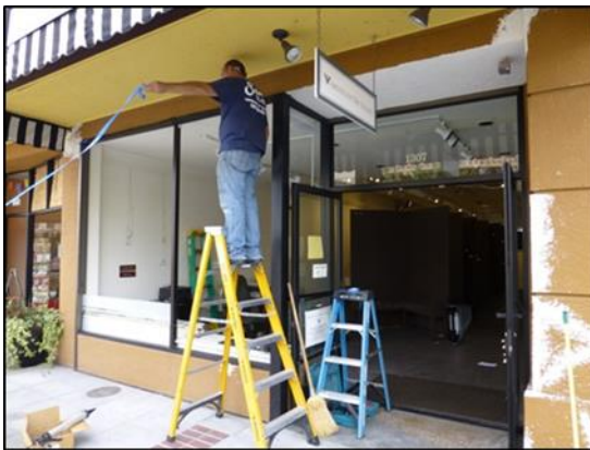
(a) Remediation of shop frontage
