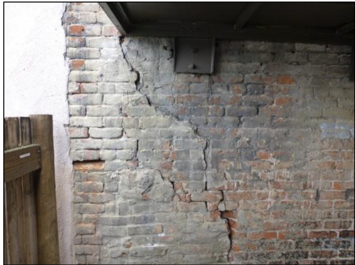
(b) Punching of walls
