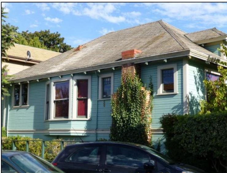
(c) Chimneys in Napa removed to roof level
