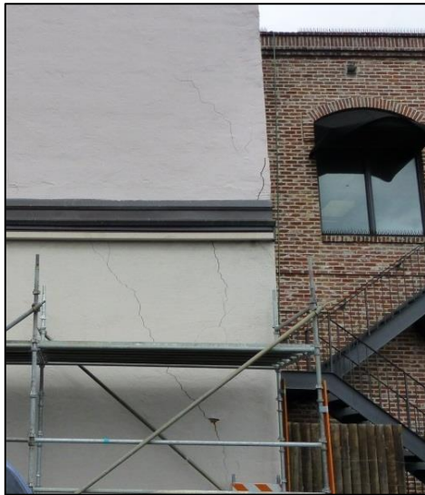
(a) Exterior stairs
