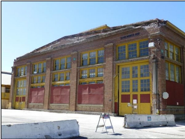
(a) Loss of parapet at the Mare Island shipyard
