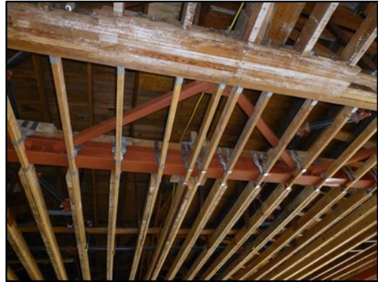
(f) Stiffening of diaphragms using steel bracing
