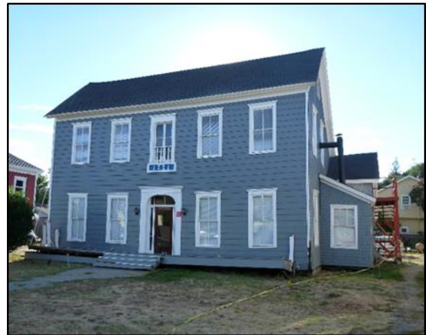
(a) Cripple wall failure in Napa
