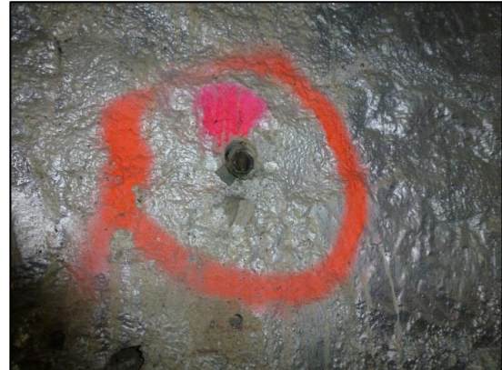
(b) Close-up of through wall anchor
