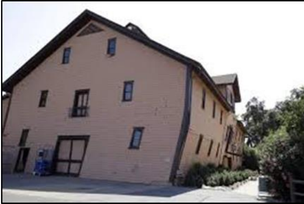
Figure 38: Timber barn at Trefethen family vineyard [65].
