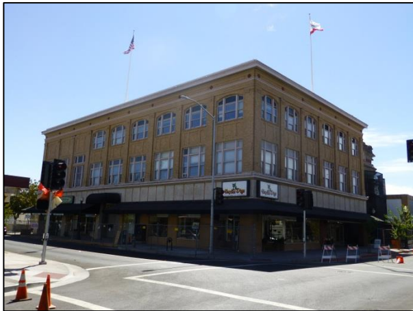
(c) A generally well-performing building
