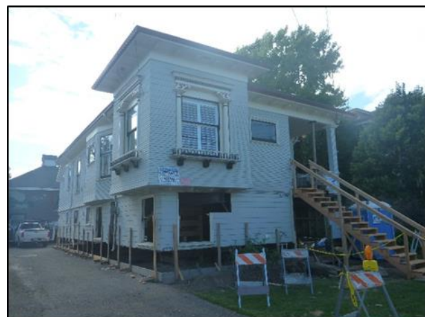
(b) House foundations under repair
