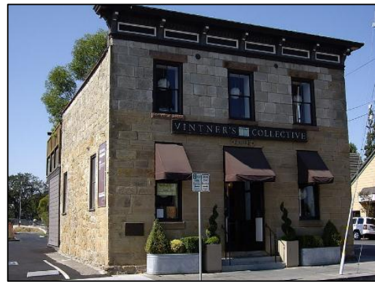
(b) 2012 condition of the building [49]
