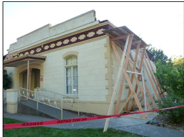
(b) Combination of props and fall protection
