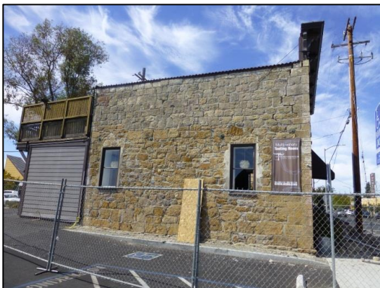
(e) Side wall showing presence of mid-height wall-diaphragm anchorages
