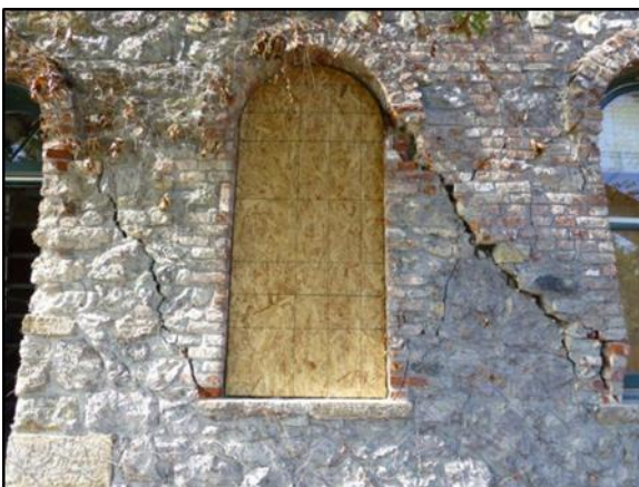
(b) Status of external repairs
