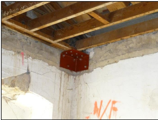
(e) Supplemental securing of diaphragm joists
