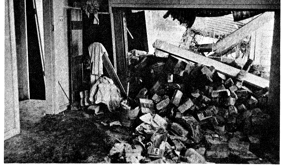
Fig. 15. Scene, kitchen, collapsed chimney and cooking stove
