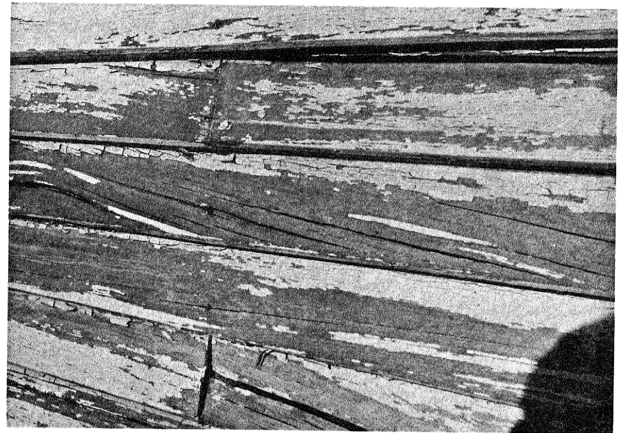
Fig. 8. Detail of view 7 at arrow, showing weather boards
