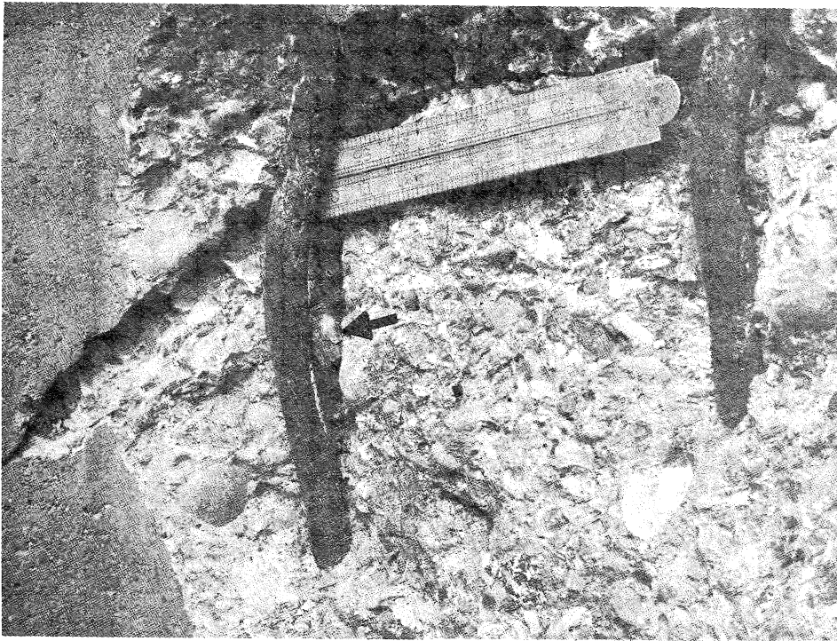
Photo 9.2: Pier 6 Detail from photo 9.1 Note the marked piece of aggregate behind the left bar. This stone fell behind the bar when it buckled and was later crushed by bar tension. The bar has since buckled again.
