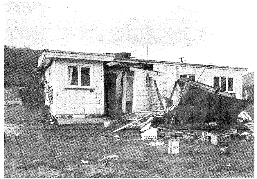
Fig. 19. Dwelling, moved, chimney collapsed, shed collapsed
