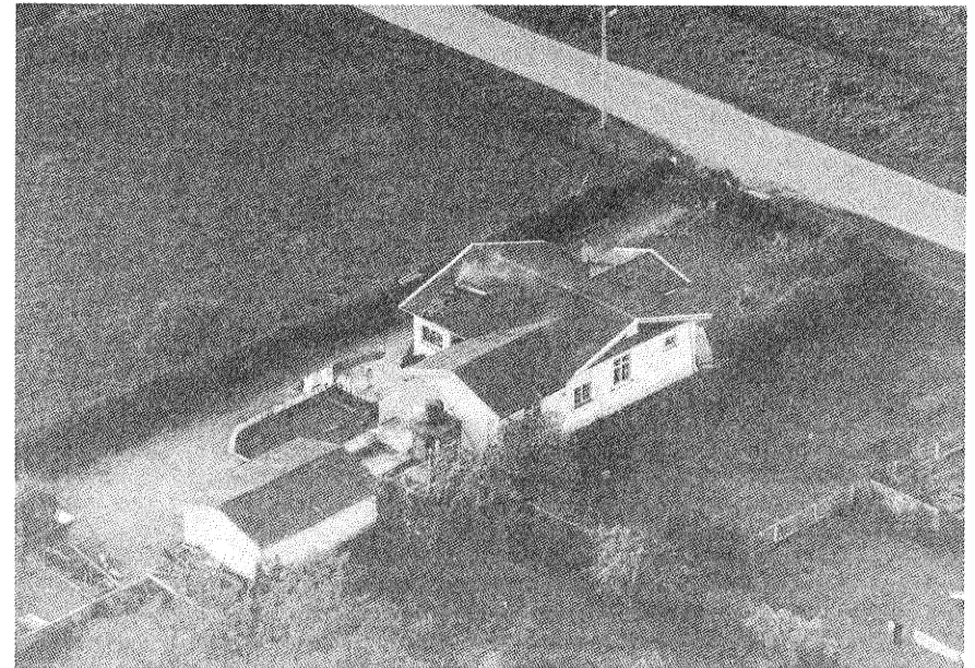
Fig. 3. Dwelling, collapsed chimney, May 24, 1968
