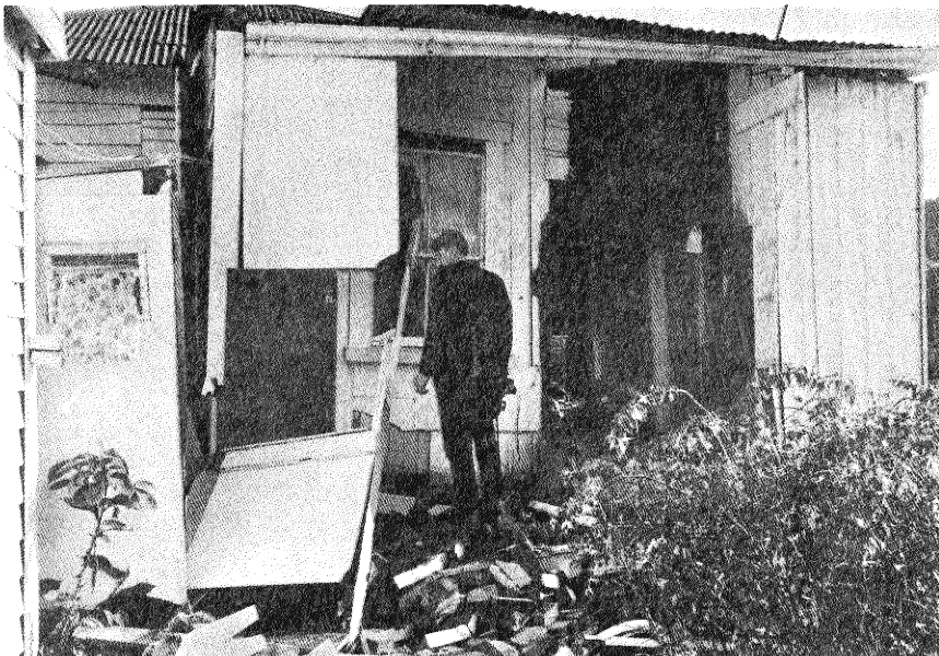
Fig. 22. rear of dwelling, fig 21
