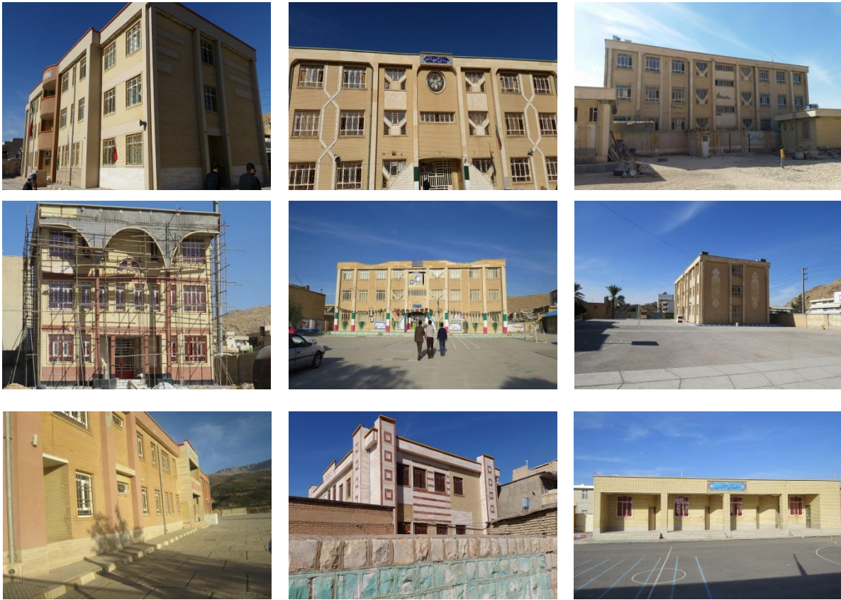
Figure 13: Steel and reinforced concrete school buildings with anchored infill walls located 10 to 40 km away from the epicenter of the earthquake.
