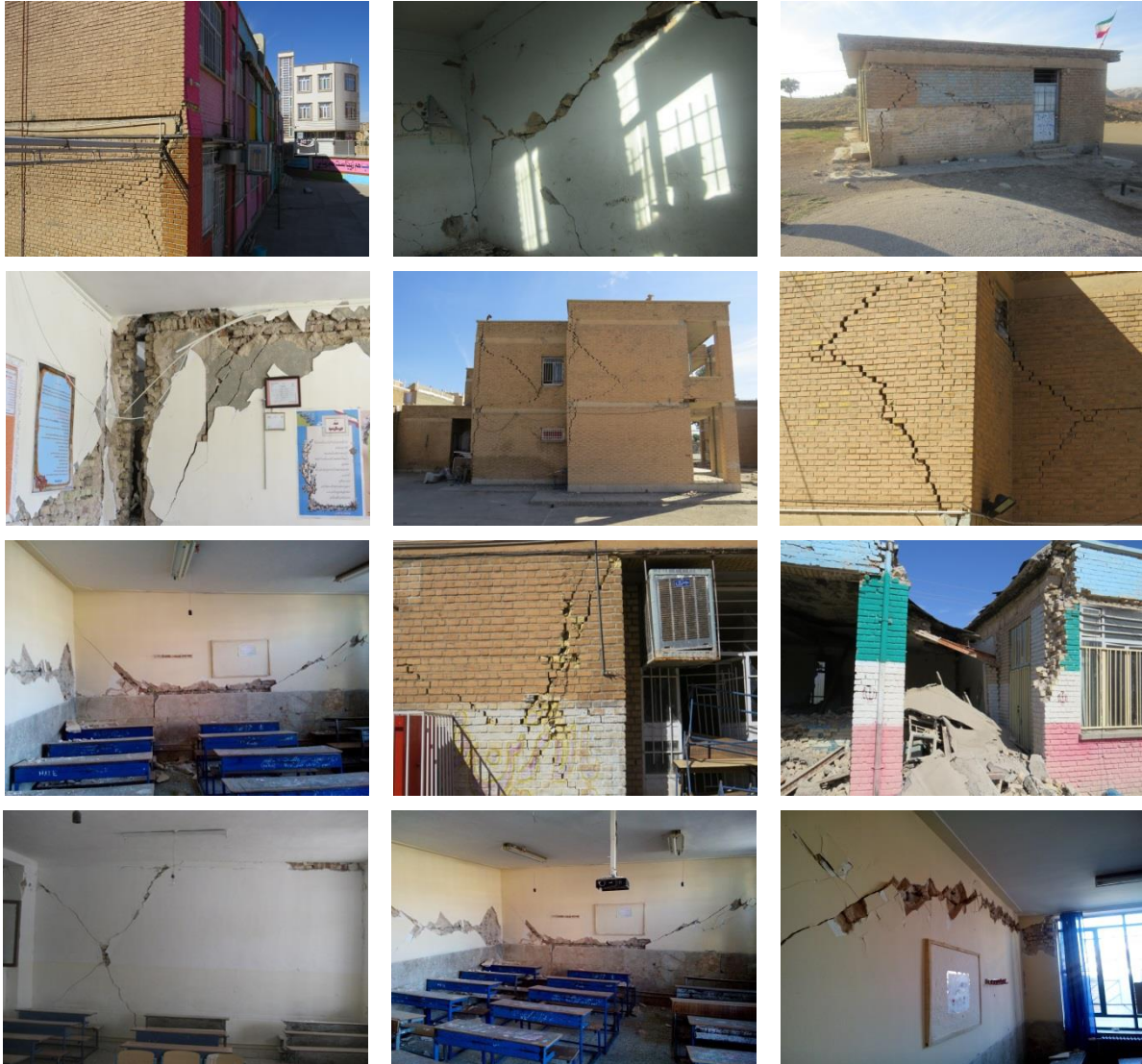
Figure 12: Damage suffered by schools located between 10 and 40 km from the epicenter of the earthquake.
