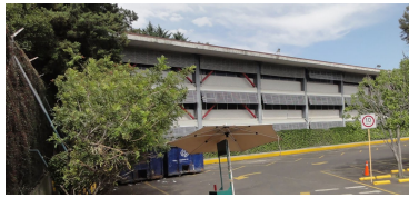
(a) No damage in the previously retrofitted high school building.
