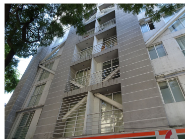
(b) Middle connection of the bracing system.
