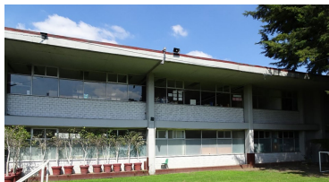
(c) No damage in the primary school retrofitted with concrete wall.
