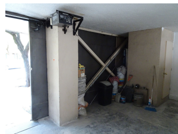
(c) Internal steel bracing in frame 3.
