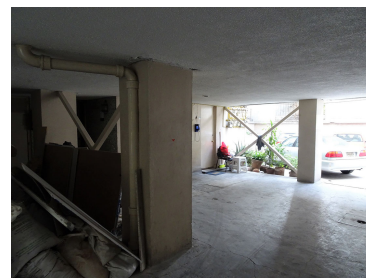
(b) Internal steel bracing in frames 1 and 2.
