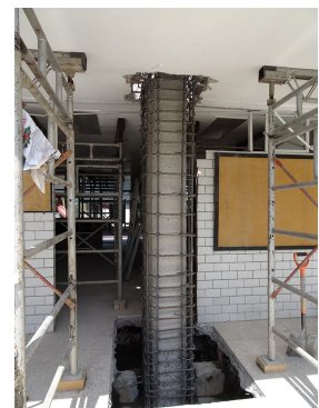
(b) Repair and retrofit of columns.
