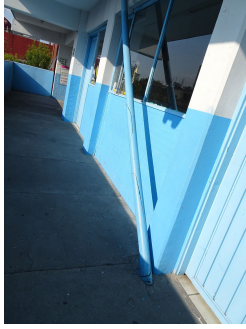
Figure 19: School building previously retrofitted with external steel braces.
