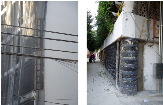
(a) Steel jacketing of box concrete columns.
