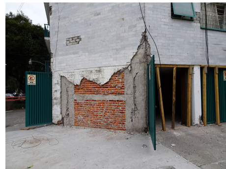
(d) View of the corner between the South and West facade.
