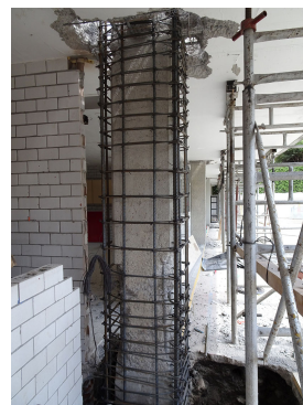
(a) Repair and retrofit of columns.
