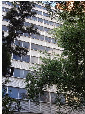
Figure 29: Steel bracing in upper levels behind the facade (building L).
