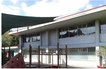
(b) No damage in the building retrofitted with concrete walls.
