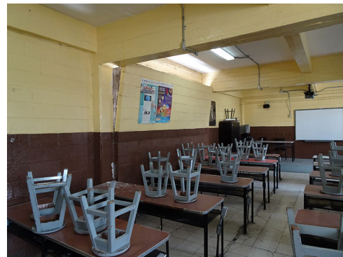
(b) Out of plane failure of the masonry wall in a school building.
