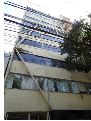
Figure 17: External bracing system.
