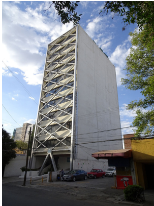
(a) Exterior steel bracing.
