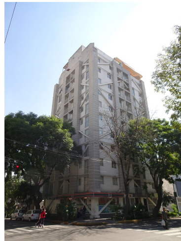
(a) North and East facades.
