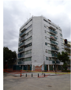
(c) Corner building to the point of collapse.
