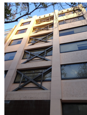
Figure 28: Building J - External bracing on the facade.
