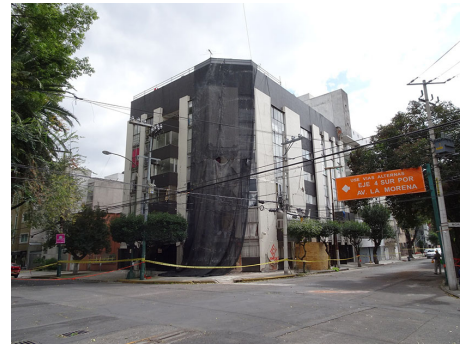
(a) Corner building heavily damaged.
