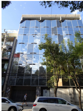
Figure 26: Building H - Glass cladding on the main facade.
