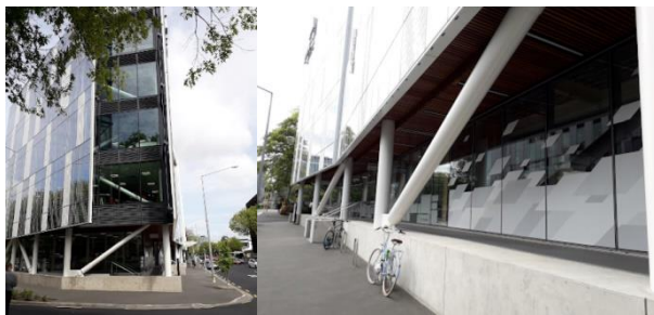
2a: Elevation 2b: Bracing system at base
