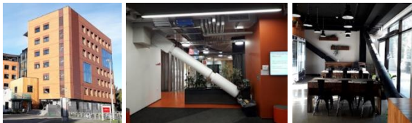
5a: Building 5b: Internal viscous damper 5c: Internal viscous dampers
