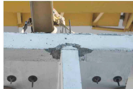
Beam-Column Connection at Second-Floor Level
