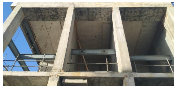
Figure 11: An apartment building in Auckland made of precast walls connected with steel beams.
