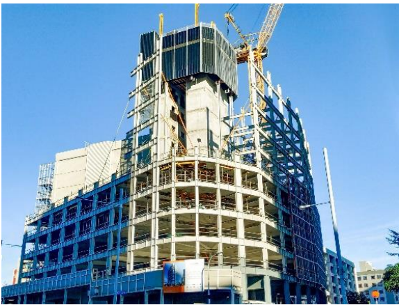
Figure 9: A hotel building in Auckland with a combined RC core with eccentrically-braced steel frames.
