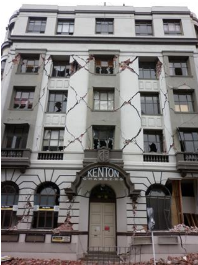
Figure 11: Examples of severe damage and collapse of masonry buildings in the CBD area, Christchurch – Lee Campbell (left, http://leelcampbell.wordpress.com ) and courtesy of Ilaria Senaldi (right).
