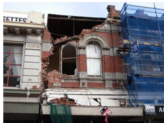
Figure 11: Examples of severe damage and collapse of masonry buildings in the CBD area, Christchurch – Lee Campbell (left, http://leelcampbell.wordpress.com ) and courtesy of Ilaria Senaldi (right).
