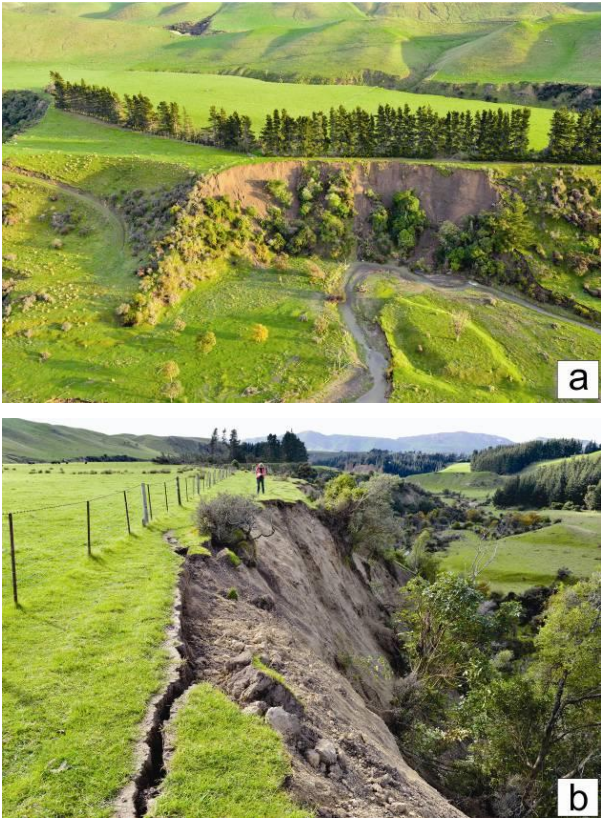
Figure 4: Landslides in the Needles Creek area triggered by the Lake Grassmere earthquake. a) Aerial view looking NNW. b) View looking ENE. (photos: D. Townsend, GNS Science; taken 2 September, 2013).
