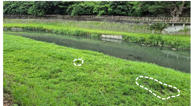
Figure 16: Localised sand boils along the banks of the Meilun river.
