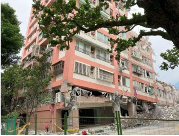
Figure 1: Demolition of a partially collapsed residential building in Hualien City.
