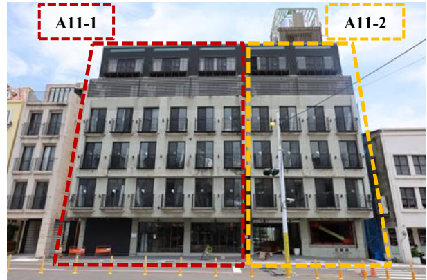
Figure 23: Building A11 with retrofitting.
