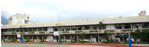
Figure 12: Building C43 with retrofitting.
