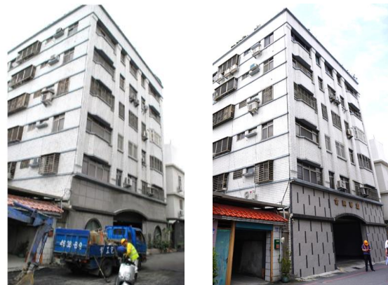
(a) Before retrofitting (a) After retrofitting
