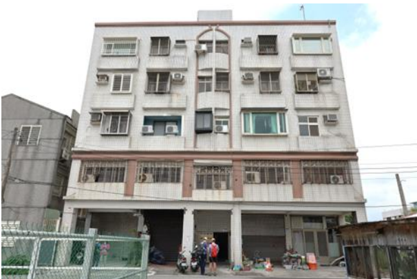
Figure 22: Building C05 without retrofitting.
