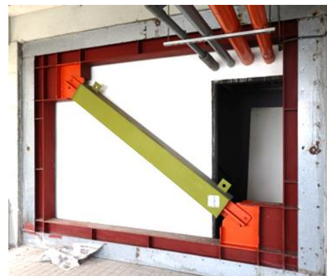
(e) Steel frame with buckling-restrained brace
