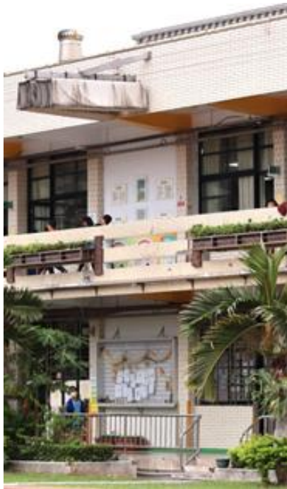
Figure 16: RC shear walls added to Building C43.
