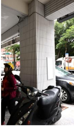
Figure 37: Exterior column with RC jacketing.
