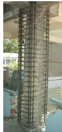
(a) RC column jacketing (Source: Chiou [3])
