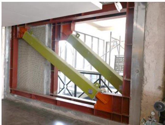
Figure 26: Steel braces added to Buildings A11-1 and A11-2.
