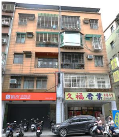
Figure 33: Building E36 with retrofitting.
