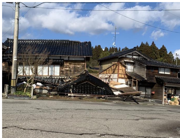
Figure 3: Typical building damage to traditional housing stock. Left hand side shows a two-storey home in which the ground floor has collapsed (soft-storey) such that the porch roof is now level with the ground. In the foreground is a single-storey home which has separated from the adjacent building to the right in a soft-storey mechanism.
