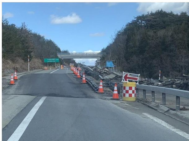
Figure 2: An example of the main highway being converted to a one-way single lane up the peninsula. A 'B-road' was utilised for the reverse direction of travel down the peninsula.
