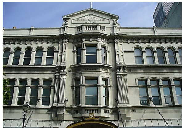
(b) Bendix Hallenstein’s Drapery and General Importing Company building (1884)
