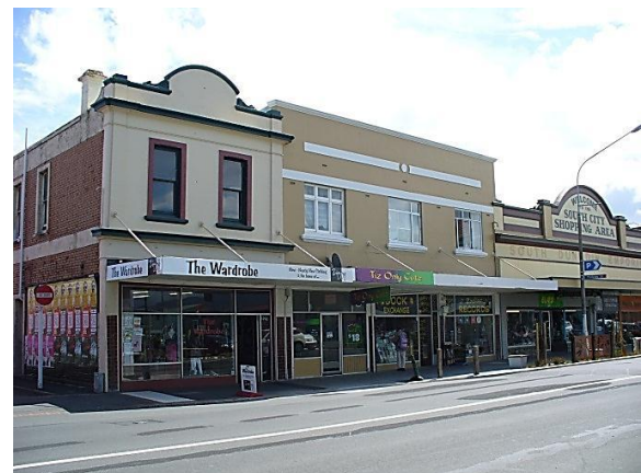
(d) URM buildings in South Dunedin.
