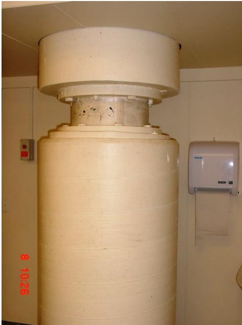
Figure 2: Left - type 1 column, showing spherical bearing in painted sleeve; Right - type 3 column in which spherical bearing is located below basement floor level near the top of the hollow casing.
