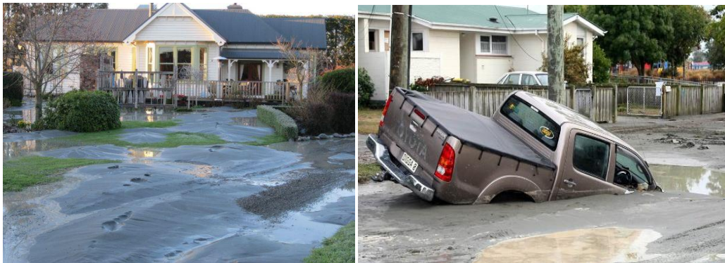
Figure 2: Examples of liquefaction in 2011 M_w 6.2 New Zealand earthquake.
