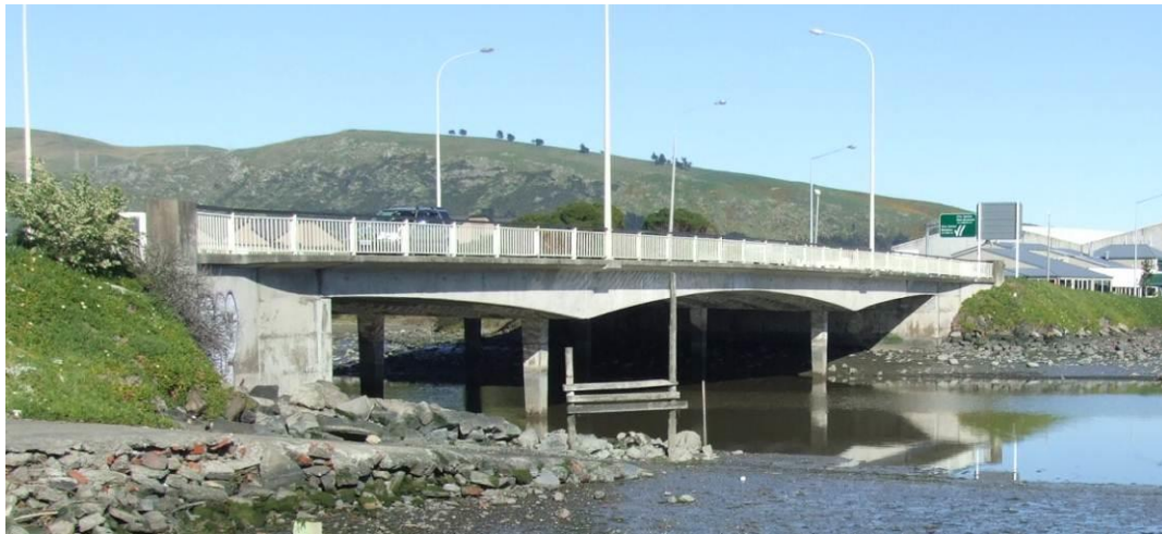
Figure 4: The recently demolished 1967 Ferrymead Bridge.
