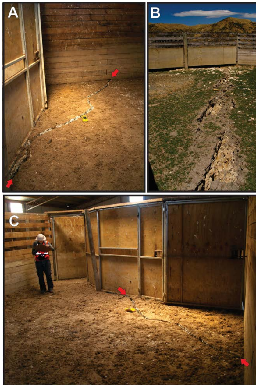
Figure 17: Mendip deer shed and northern Leader Fault surface rupture; see Figures 1 & 18 for location (Lat: -42.5740 , Long: 173.2825 ). (A), (B), & (C) Field photographs of normal faulting running through the deer shed. (B) is looking to the southeast, across the stock yard and towards the intersection of the two fault sets (see text for discussion). Photos taken by Clark Fenton in January 2017.
