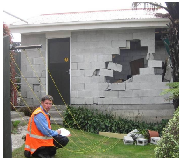
Figure 38: UngROUTED cells with reinforcing steel in place (Beattie).
