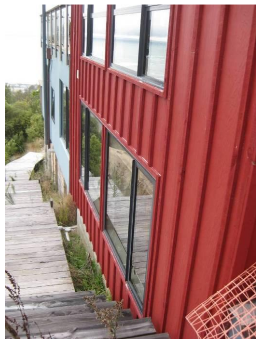
Figure 11: Plywood sheet cladding with timber battens (Beattie).
