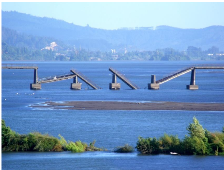
Figure 8.5: Collapsed bridge across Bio-Bio River. (Courtesy of A. García).
