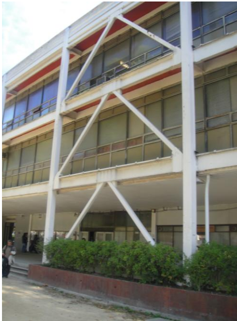
Steel K braced retrofitted to three-storey building at University of Concepción.
