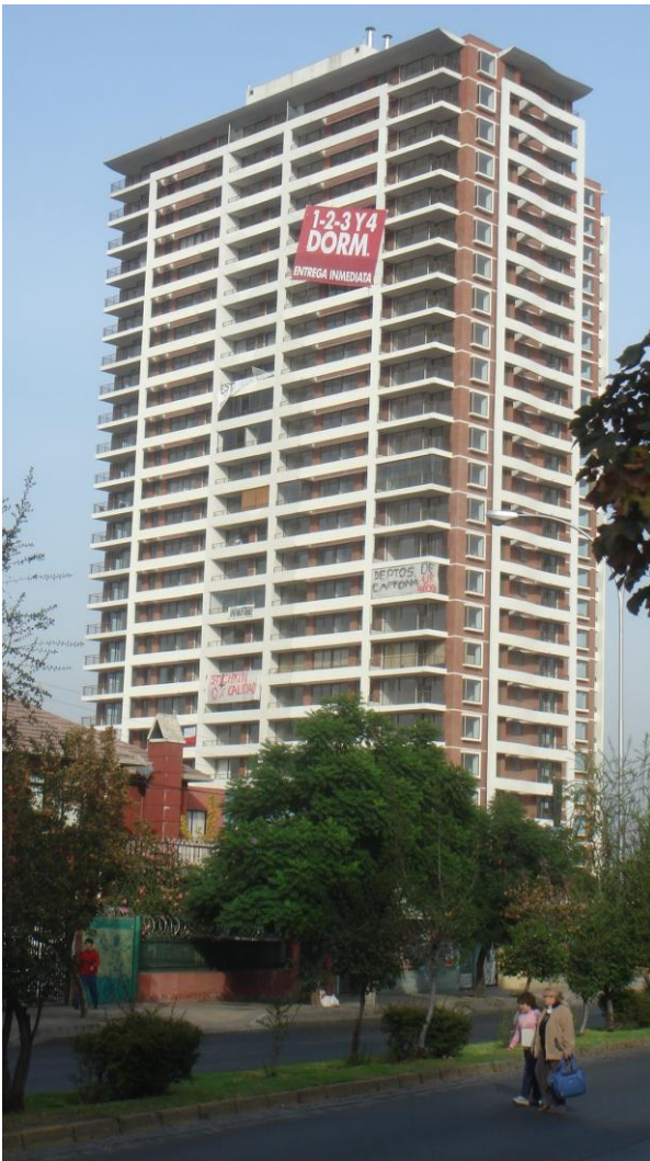
Los Cerezos Apartment building in Santiago.
