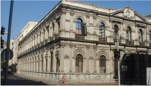
Temporary support of Building façade in central Santiago.
