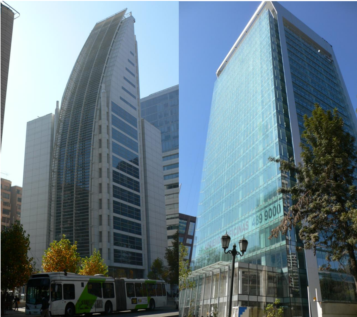
Figure 5.9b: Examples of curtain wall glazing that survived the earthquake with no damage in Santiago. (Photos: Graeme Beattie).
