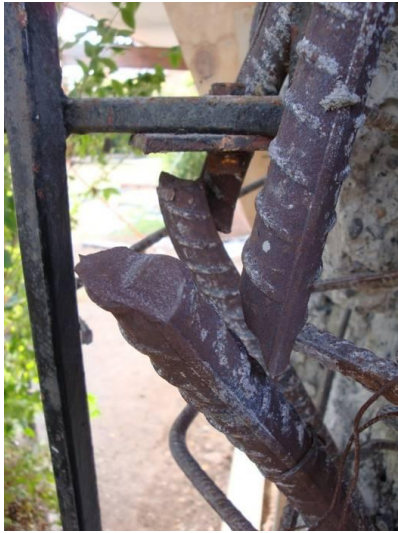
Figure 5.3g and 5.3h: Fractured reinforcing steel in single storey reinforced concrete frame (left) and damaged shear wall (right). (Photos: Clark Hyland).
