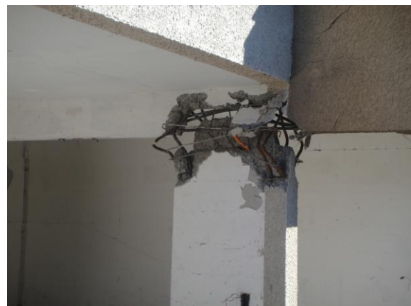
Figure 5.3i: Shear wall failures, Plaza del Rio, Concepción. (Photos: Peter Smith).
