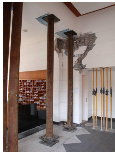
Figure 5.3: (c - left) Collapse of a shear wall in a multi-storey apartment block in Viña del Mar. (d - right) Use of temporary props in another damaged apartment block. (Photo: Graeme Beattie).
