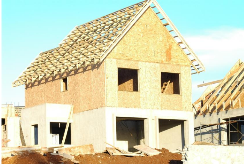
Figure 5.1c: Residential home in Concepción incorporating lower storey of reinforced masonry and upper storey of plywood and timber frame. (Photo: Hugh Cowan).
