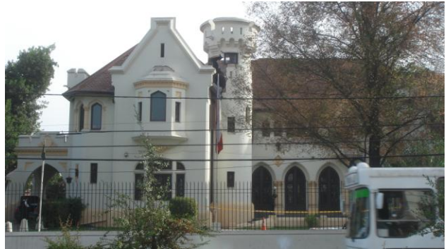
Pounding between tower and dwelling in Santiago.
