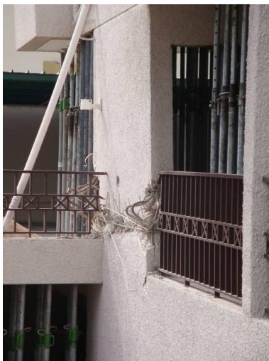
Figure 5.3: (c - left) Collapse of a shear wall in a multi-storey apartment block in Viña del Mar. (d - right) Use of temporary props in another damaged apartment block. (Photo: Graeme Beattie).
