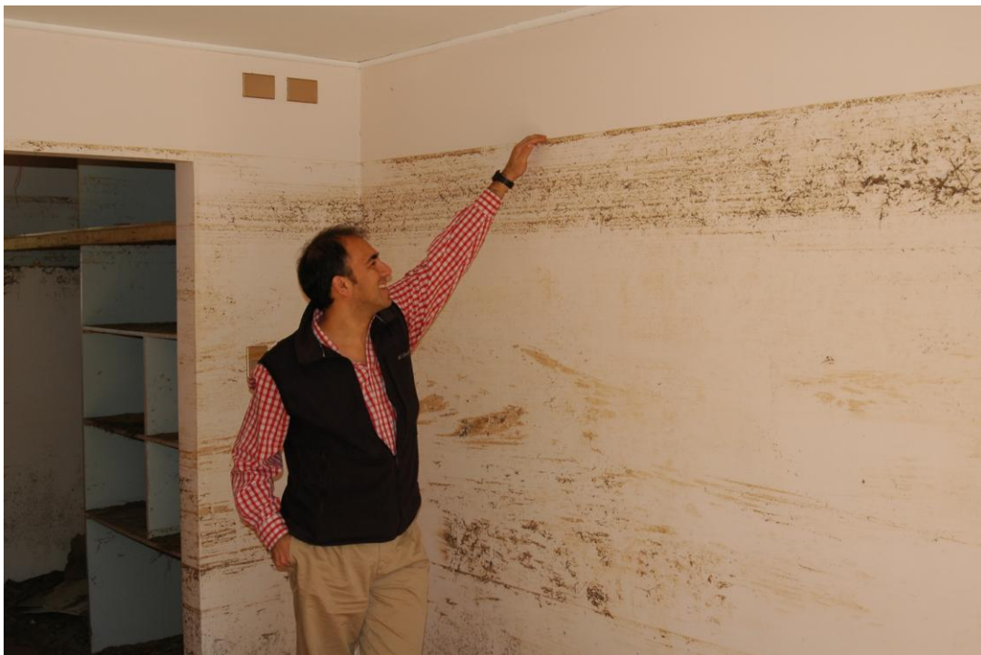
Figure 2.2b: Tsunami fill-depth of ~2 m in homes at the coastal resort of El Pingueral, north of Concepción. (Photo: Hugh Cowan).
