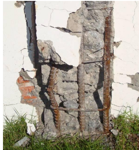
Figure 5.3g and 5.3h: Fractured reinforcing steel in single storey reinforced concrete frame (left) and damaged shear wall (right). (Photos: Clark Hyland).
