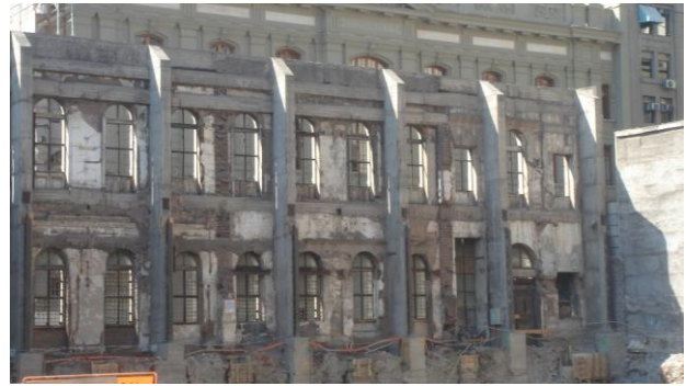
Temporary support of Building façade in central Santiago.
