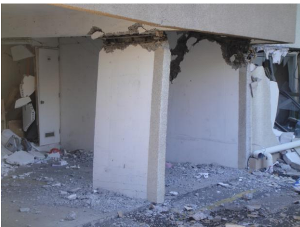
Figure 5.3i: Shear wall failures, Plaza del Rio, Concepción. (Photos: Peter Smith).
