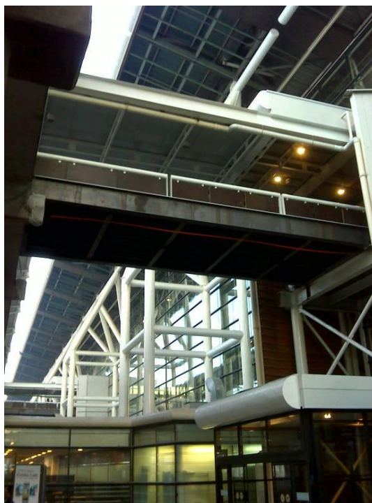
Figure 8.6: Replaced linkspan from access roadway to terminal. (Photo: Graeme Beattie).
