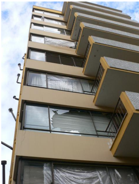
Figure 5.9a: Examples of buildings in Concepción with broken exterior glazing. (Photos: Graeme Beattie).
