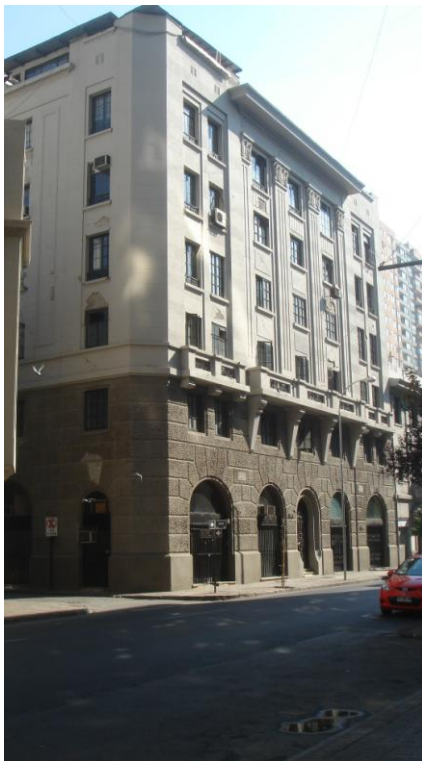
Damaged spandrels to early reinforced concrete building in central Santiago.
