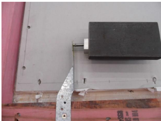
(d) Complete detachment of sheets, showing slotting and head pull through
