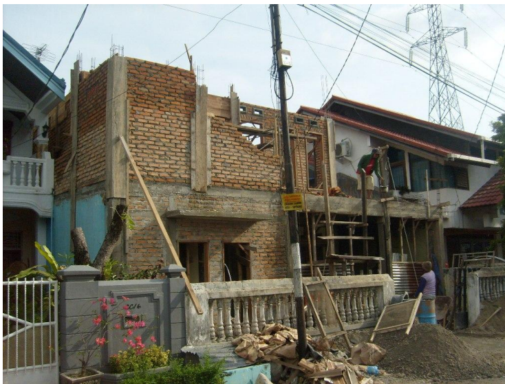
b) A brick masonry building under construction.
