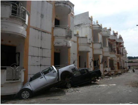
Figure 6.1: Several examples of soft storey failure.
