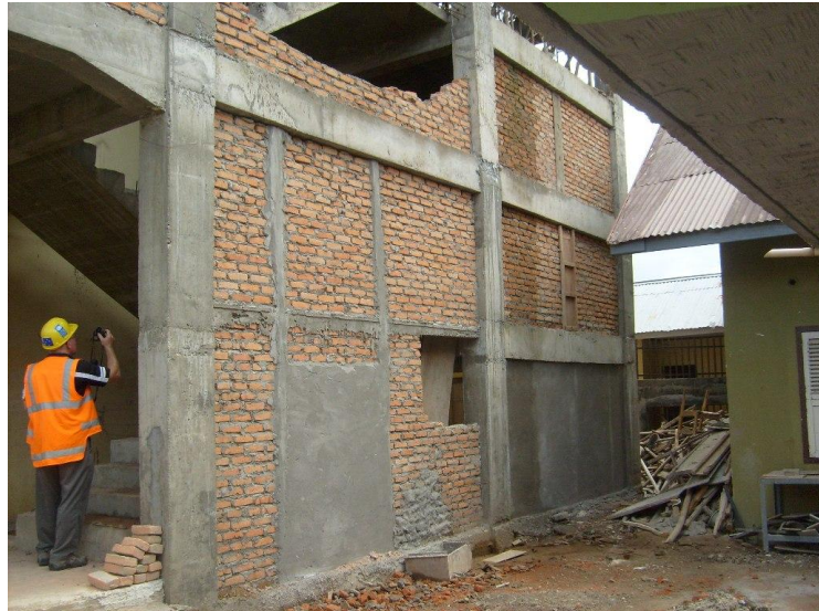
a) Brick infill panels with practical columns and beams.
