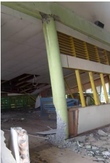
Figure 6.21: Excellent performance of a column with spiral stirrups in the bus terminal building.
