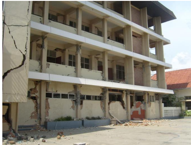
a) Plastic hinges distributed along the height of the building, presumably due to the similar strength and stiffness of each level.
