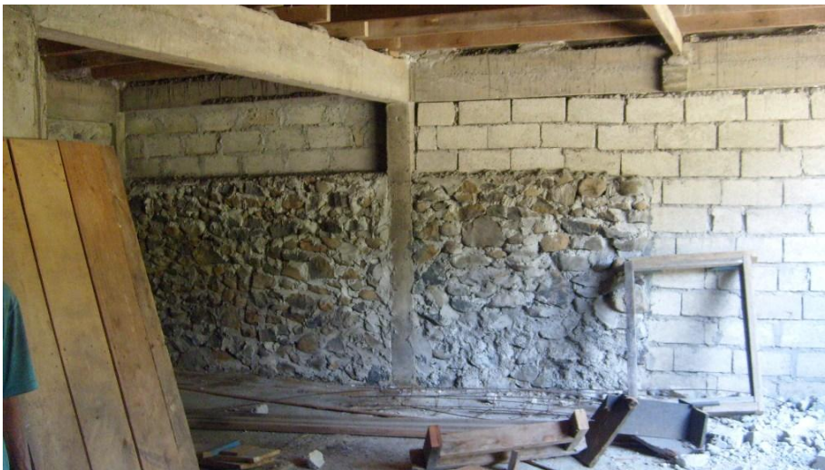
b) Mixing of infill wall materials.
