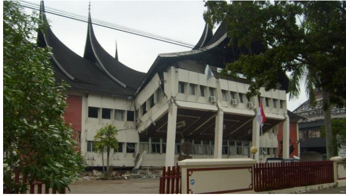
Figure 6.1: Several examples of soft storey failure.
