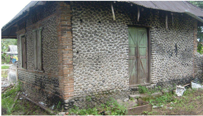
Figure 6.15: A stone masonry building with unreinforced brick columns.
