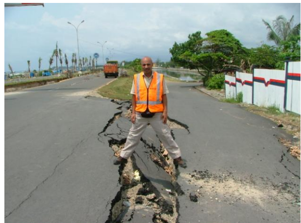
Figure 3.3: Lateral spreading and settlement of the present-day beach ridge. The ocean is to the left and a lagoon area to the right.
