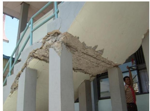
b) Close-up view of staircase in (a).
