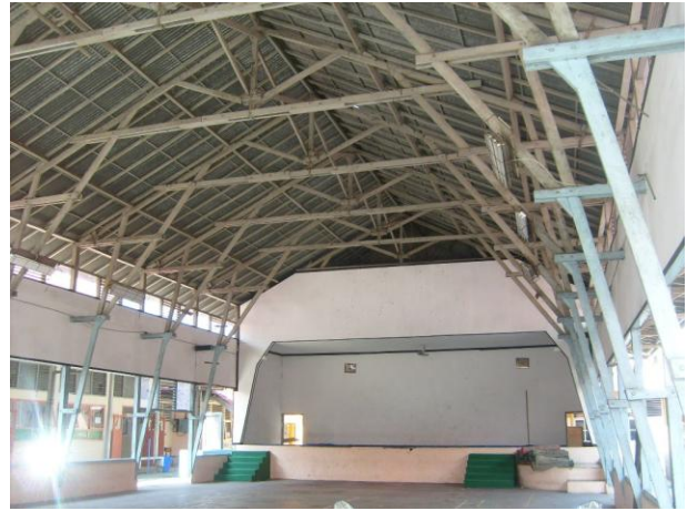
b) A large span timber frame structure without any damage.
