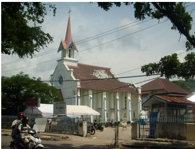
Figure 6.14: Church with undamaged bell tower.
