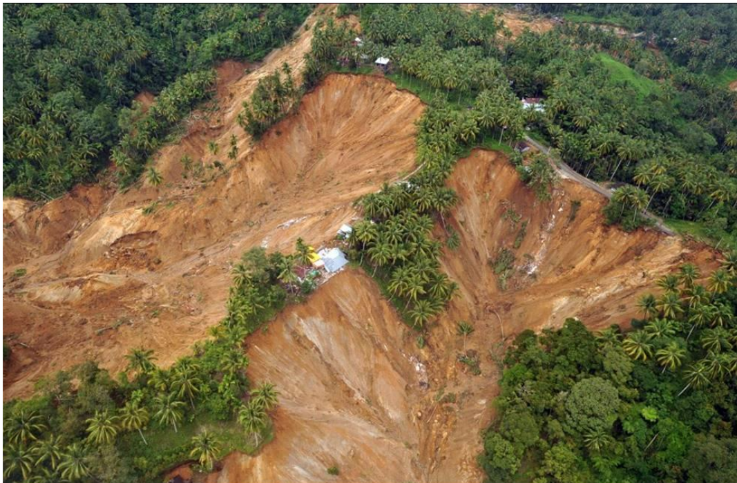
Figure 3.8: Slope failures in volcanic tuffs some 70 m deep triggered by the earthquake. These unexpected earth flows from moderately steep slopes buried several villages and killed more than 600 people.
