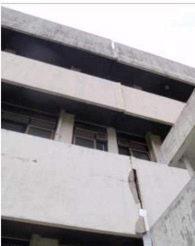
Figure 6.4: Pounding damage.
