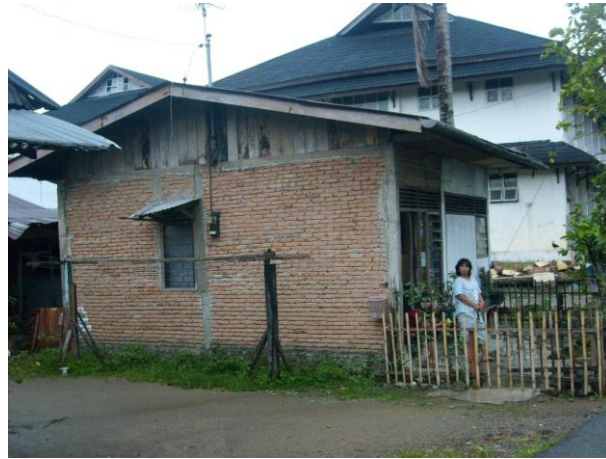
a) A typical brick masonry building in the area.
