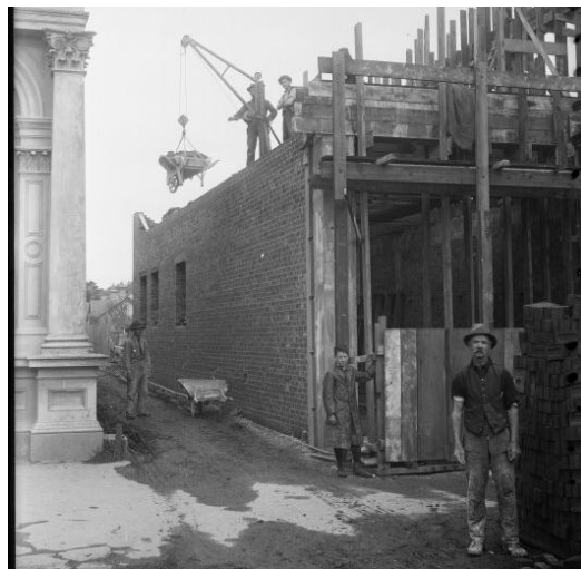
Figure 8: Brick building under construction, ca. 1920 [Alexander Turnbull Library].
