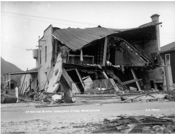
Figure 15: General store damaged by the 1929 Murchison earthquake [Alexander Turnbull Library].
