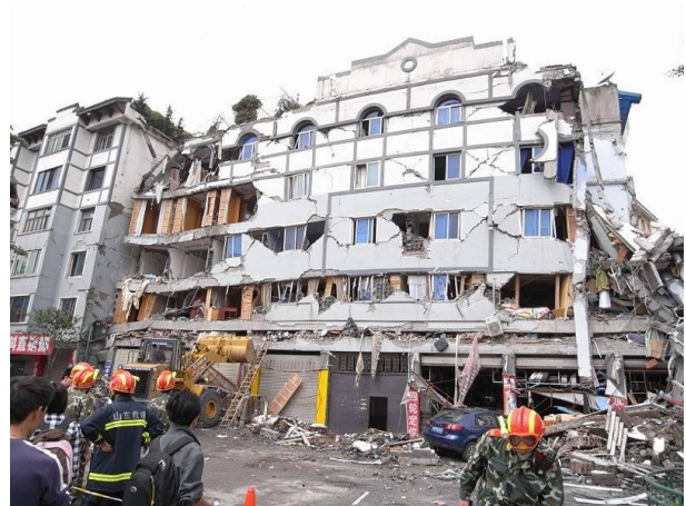
Figure 67: Collapse of an entire floor in Dujiangyan (MM X), Type 2 Masonry Construction.
