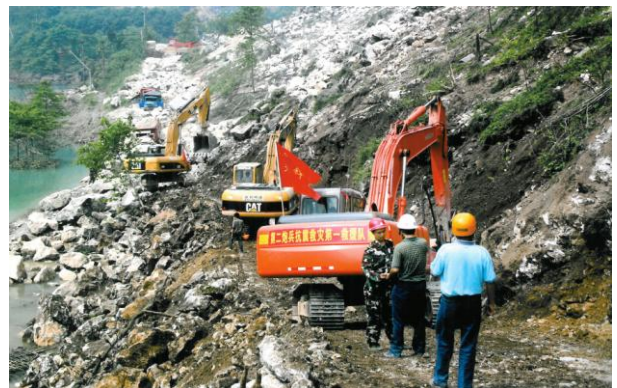
Figure 139: Reinstating access along roads closed by landslides.
