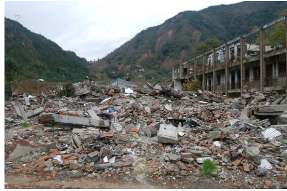
Figure 72: Beichuan school building totally collapsed - URM construction.
