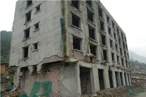
Figure 52: Type 2 Masonry Structure: Hybrid with reinforced concrete structure at the bottom level and URM above. Note the complete failure of the URM floor.
