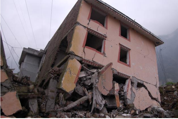
Figure 51: Type 1 Masonry Construction in Yingxiu, complete collapse.
