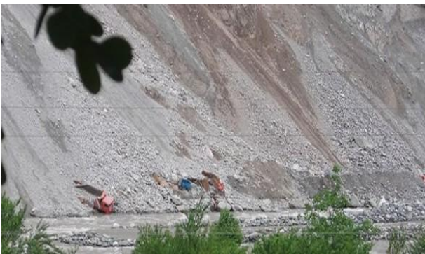
Figure 126: Highway completely removed by landslides.
