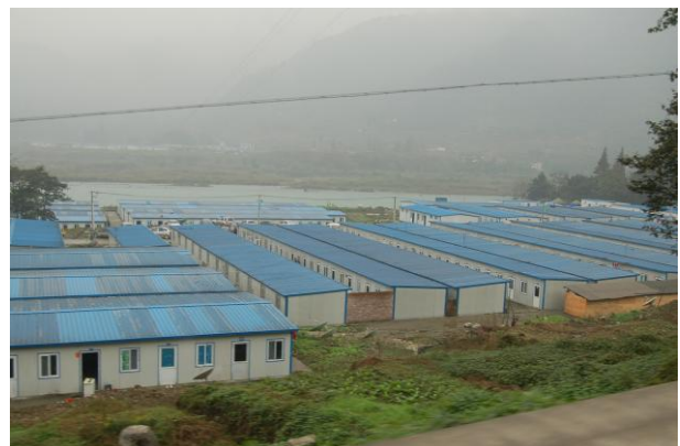
Figure 143: A temporary housing village.
