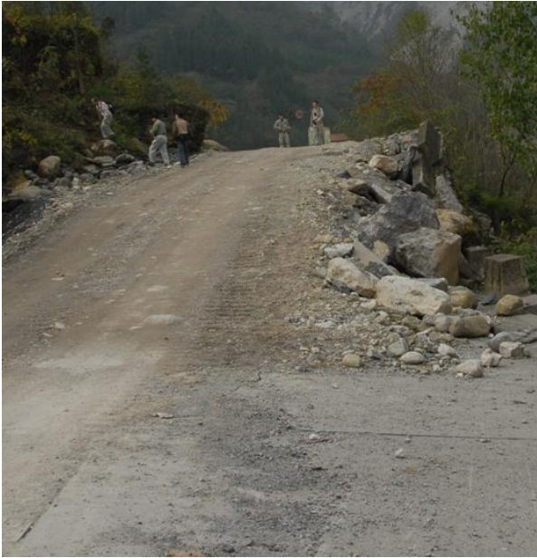
Figure 21: The displacement of the Yingxiu-Beichuan fault near Qingping Village. The vertical displacement is of ~4 m.
