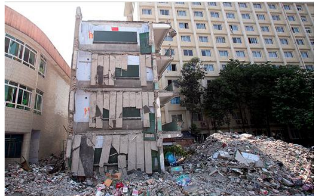
Figure 68: Collapse of a school building in Dujiangyan (MM X). Note the precast hollowcore floor units hanging with no topping and no tie bars.
