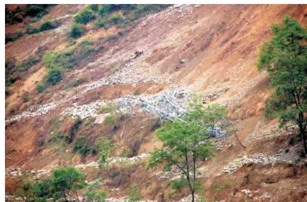
Figure 120: Transmission tower destroyed by landslide.
