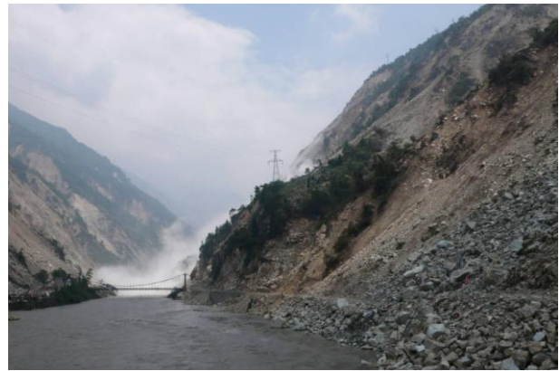
Figure 138: Highway completely removed by landslides.
