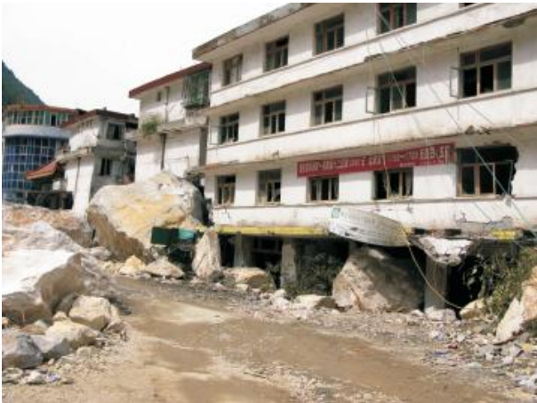
Figure 109: Buildings damaged by large rock boulders.
