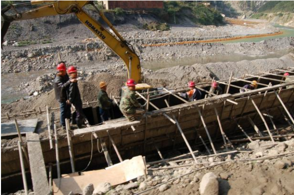
Figure 114: Reconstruction of gravity retaining wall to replace walls that had collapsed.
