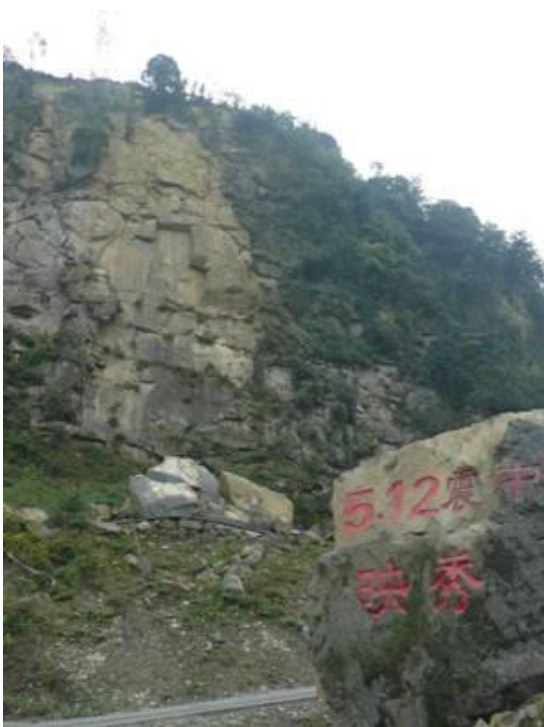
Figure 37: Rockfall from slope near Yingxiu. Rockfall is a symbolic epicentral marker.
