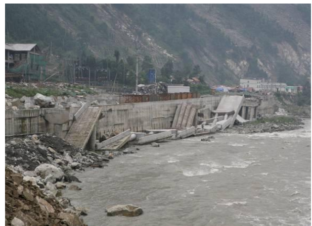
Figure 92: Complete collapse of a bridge across the fault rupture at Yingxiu near the epicentre.
