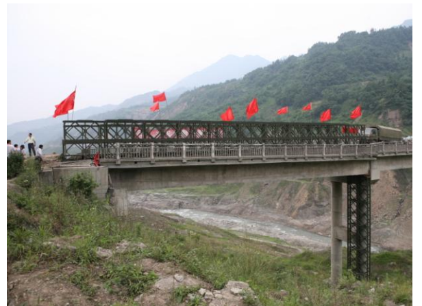
Figure 134: Reinstating temporary access across damaged bridges using truss structures.
