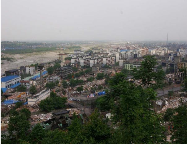
Figure 63: Hanwang township - note the collapse of the buildings.
