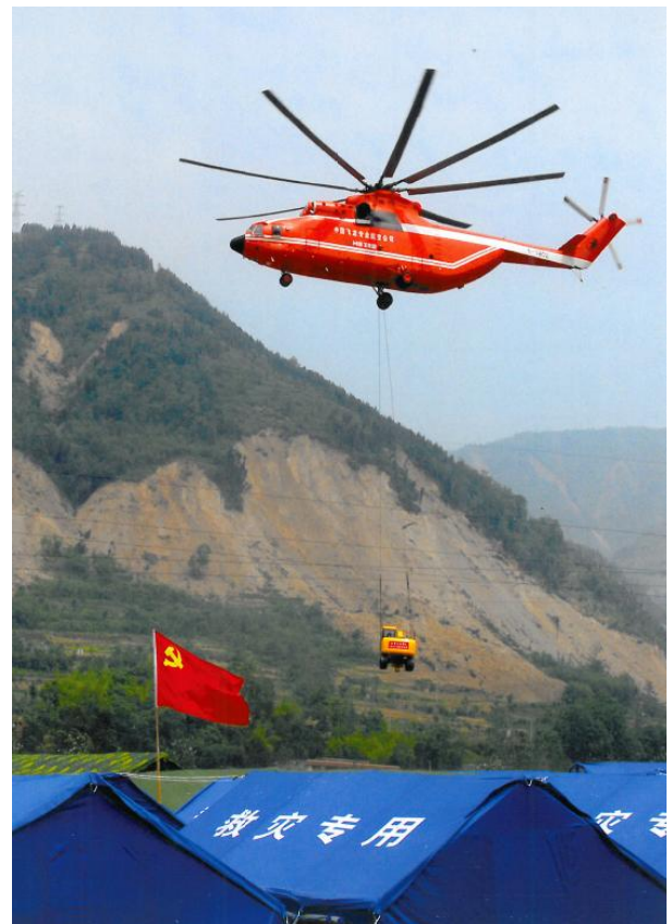
Figure 140: Transport of heavy plant by helicopter.
