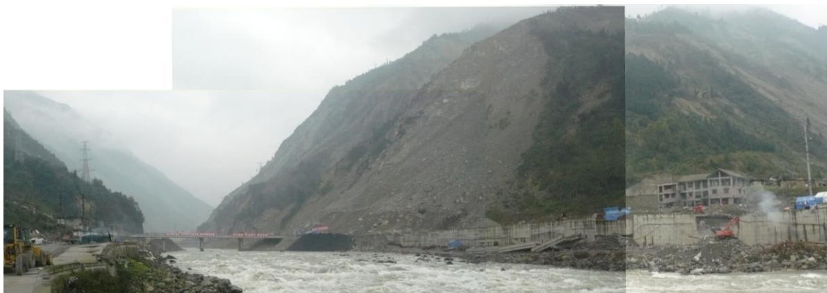
Figure 43: Fault scarp and deep seated landslide at Yingxiu. Rapids formed by the vertical fault offset (Figure 15) and the bridge over Minjiang River made serviceable after being skewed off piers when hit by the landslide. The bridge structure alongside the river on the other bank was also completely destroyed, (Figures 92 & 93).
