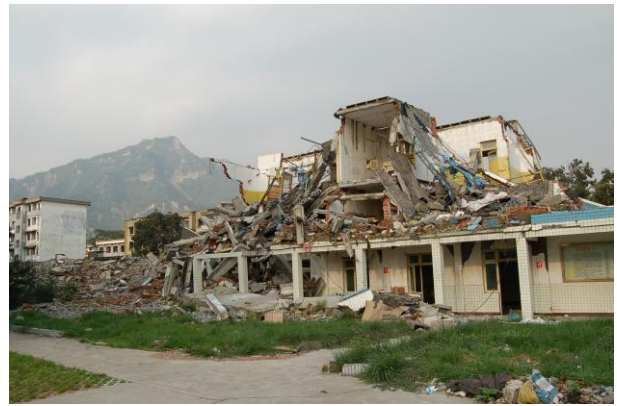
Figure 66: Mianzhu No.3 Hospital in Hanwang township – near complete collapse.
