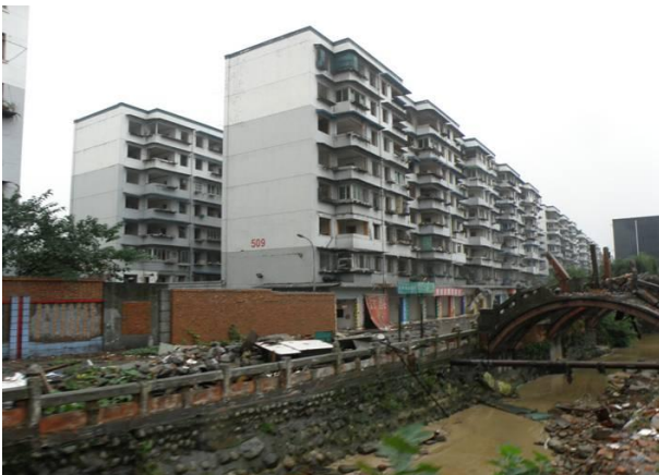
Figure 65: Hanwang township, these buildings survived and performed relatively well.
