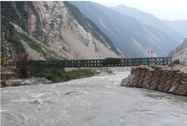
Figure 135: Reinstating temporary access across rivers using truss bridges.
