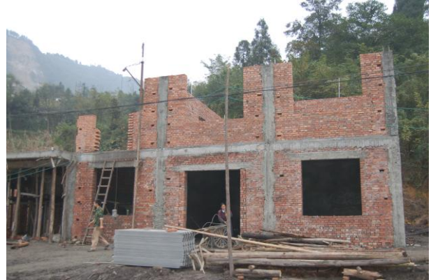
Figure 147: Reconstruction of houses, typically in masonry.
