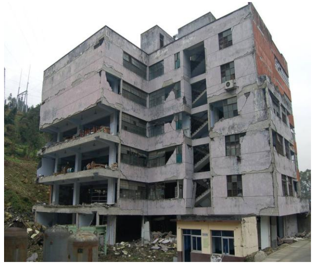
Figure 54: Shear wall building in Yingxiu; good performance observed.
