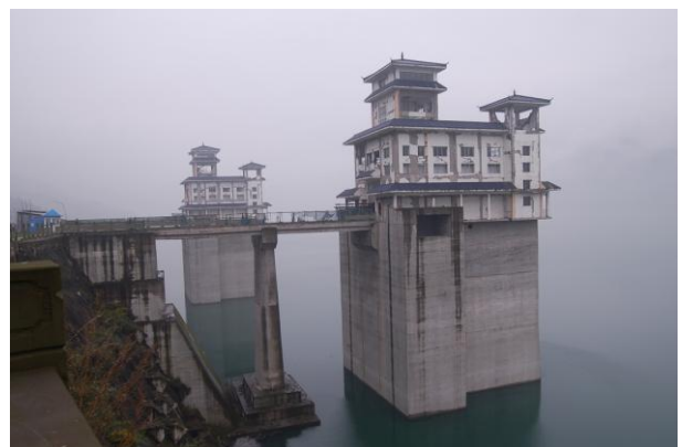
Figure 101: Intake structures low level outlet tunnels. Some damage to tower superstructures is apparent, but tunnels operated after earthquake.
