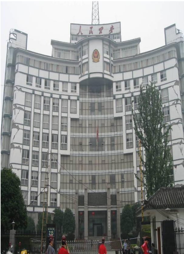
Figure 74: Public Security Bureau in Dujiangyan (MMX), some structural damage but intact, reinforced concrete frame - shear wall structure.
