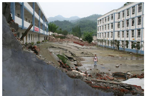
Figure 24: The Peng-Guan fault rupture in the Bailu School campus. The vertical displacement was ~2 m. Two buildings used to sit on top of the fault line were brought down by fault rupturing and only ruins were visible in the frontal and distal parts of the photo.
