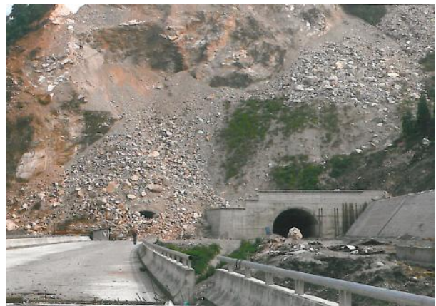
Figure 117: Tunnel portal blocked by rock slides.
