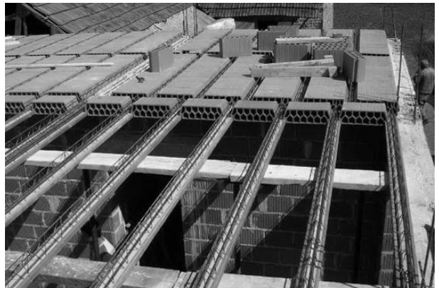
Figure 16: Photo of perforated masonry diaphragm system (courtesy of Sanja Hak).
