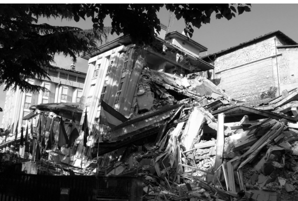
Figure 14: Collapsed R/C frame building (L'Aquila).
