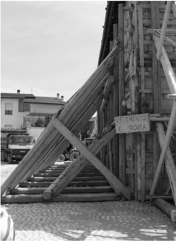
Figure 19: Propped structure to prevent the collapse of masonry wall (Onna).
