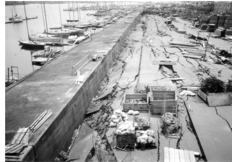
Figure 2: Failure of backfill ground behind gravity quay wall (Nishinomiya Harbour).
