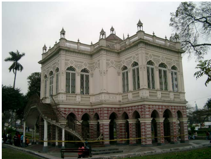
Figure 44. Undamaged building Lima
