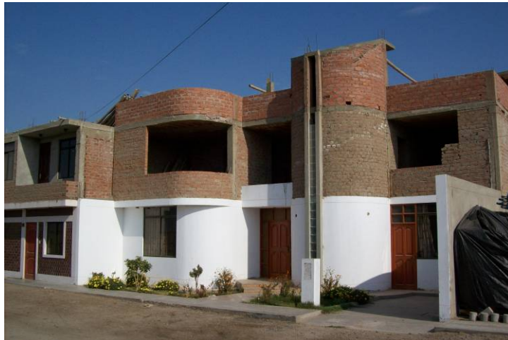
Figure 62. Undamaged Engineered Confined Masonry Dwelling - Pisco
