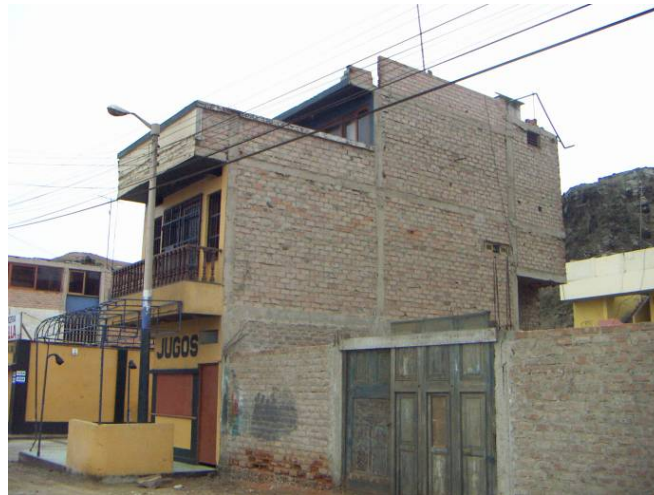
Figure 36. Confined Masonry Building
