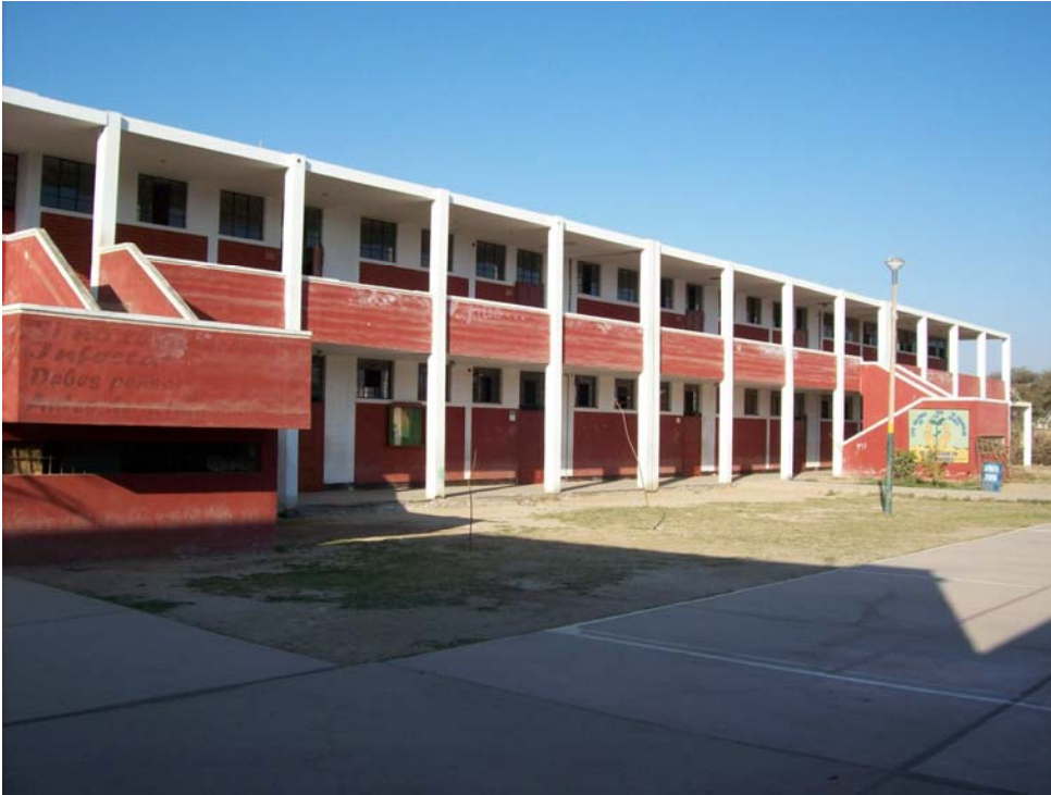
Figure 86. Undamaged school – Ica
