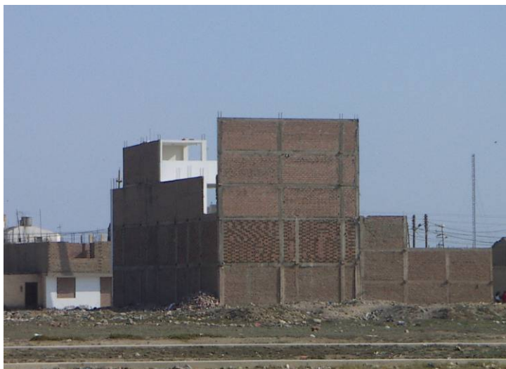
Figure 63. Multistorey Confined Masonry Building - Pisco
