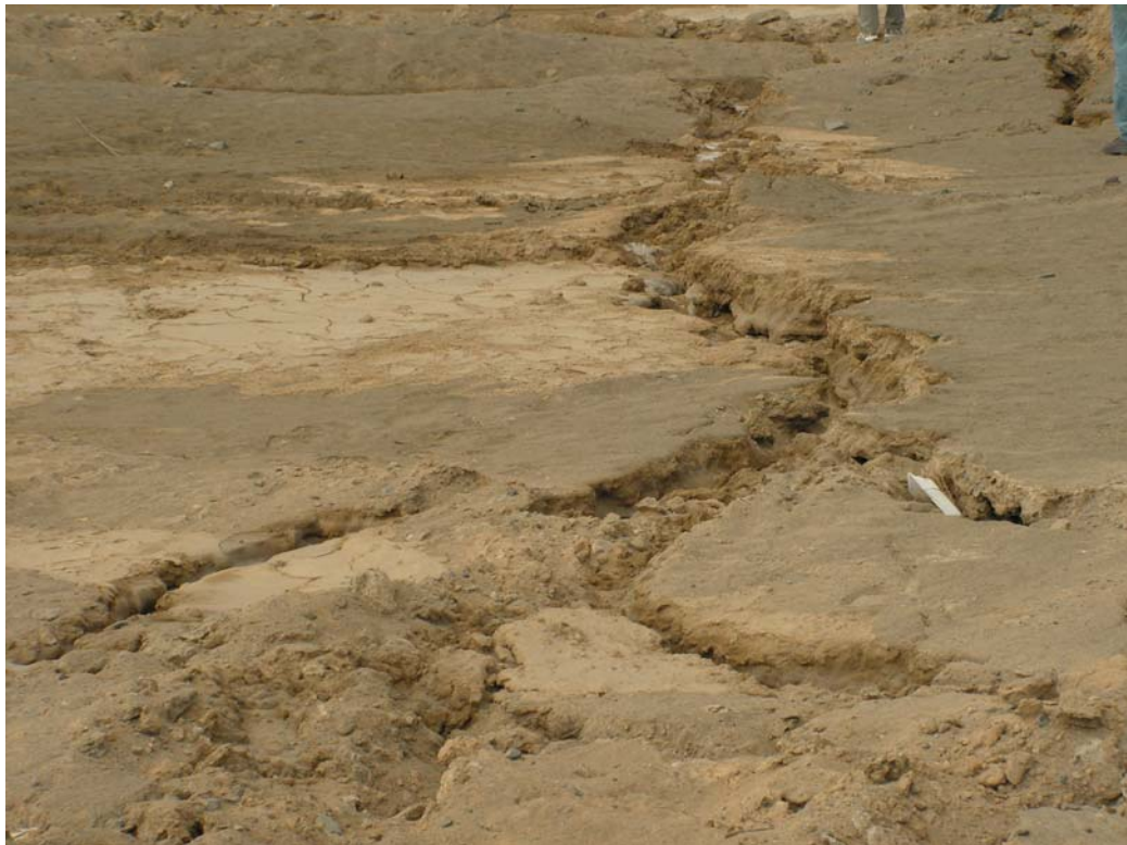
Figure 26. Surface cracking from liquefaction
