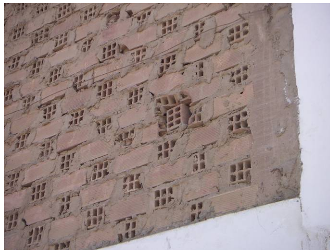
Figure 37. Infill Masonry Brick
