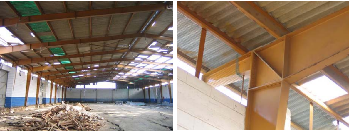
Figure 99. Steel Portal Warehouse, Port of San Martin
