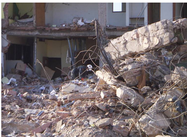
Figure 70. Demolished Embassy Hotel – Pisco
