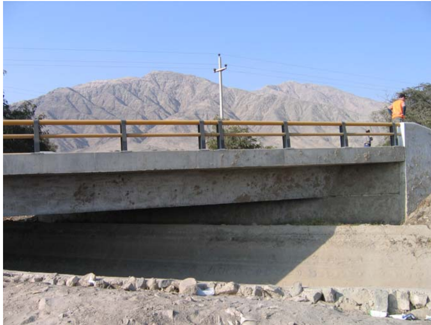
Figure 103. Typical bridge on Carretera los Libertadores (Route 24a)
