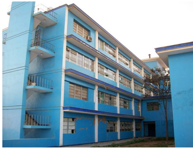
Figure 88. Regional Hospital – Ica
