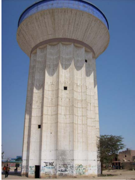
Figure 116. 1,200 cubic metre reservoir in Ica
