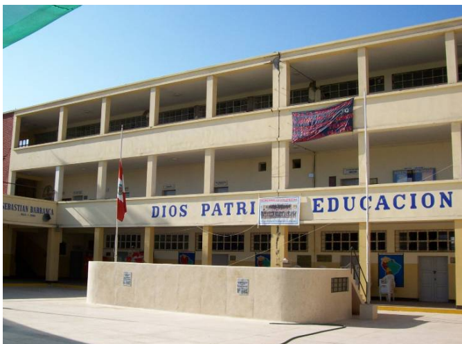
Figure 79. Damaged School - Ica
