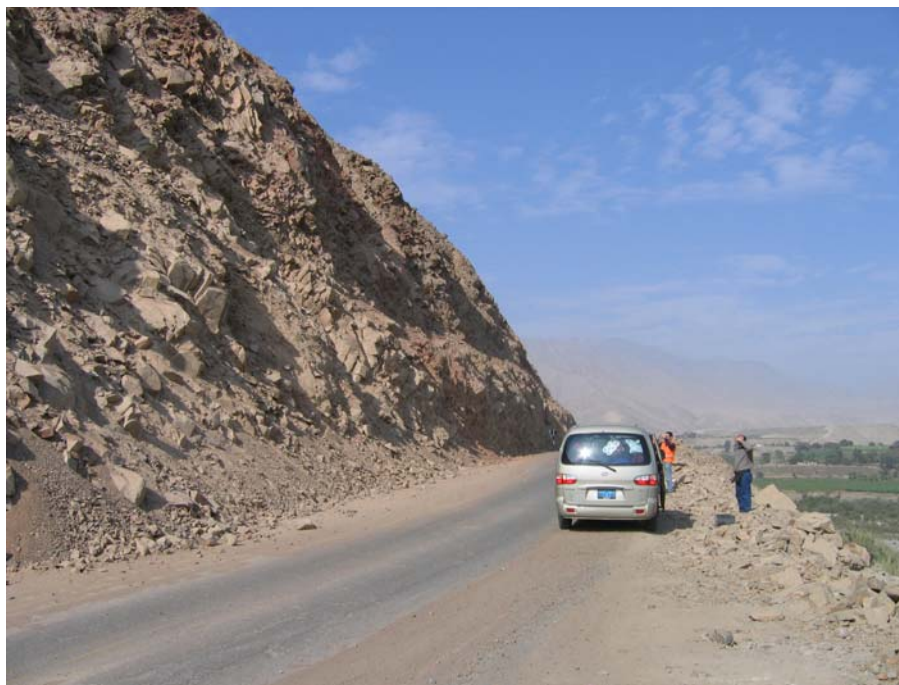
Figure 107. Rock falls on Route 24a
