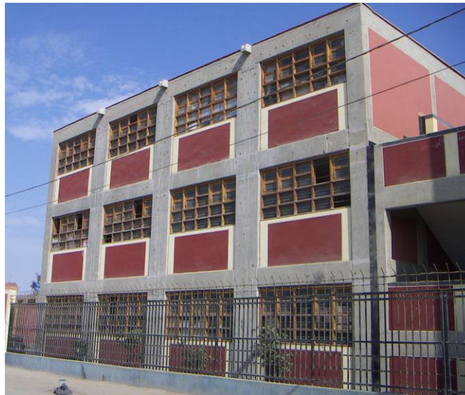
Figure 82. School Constructed to New Standard - Pisco
