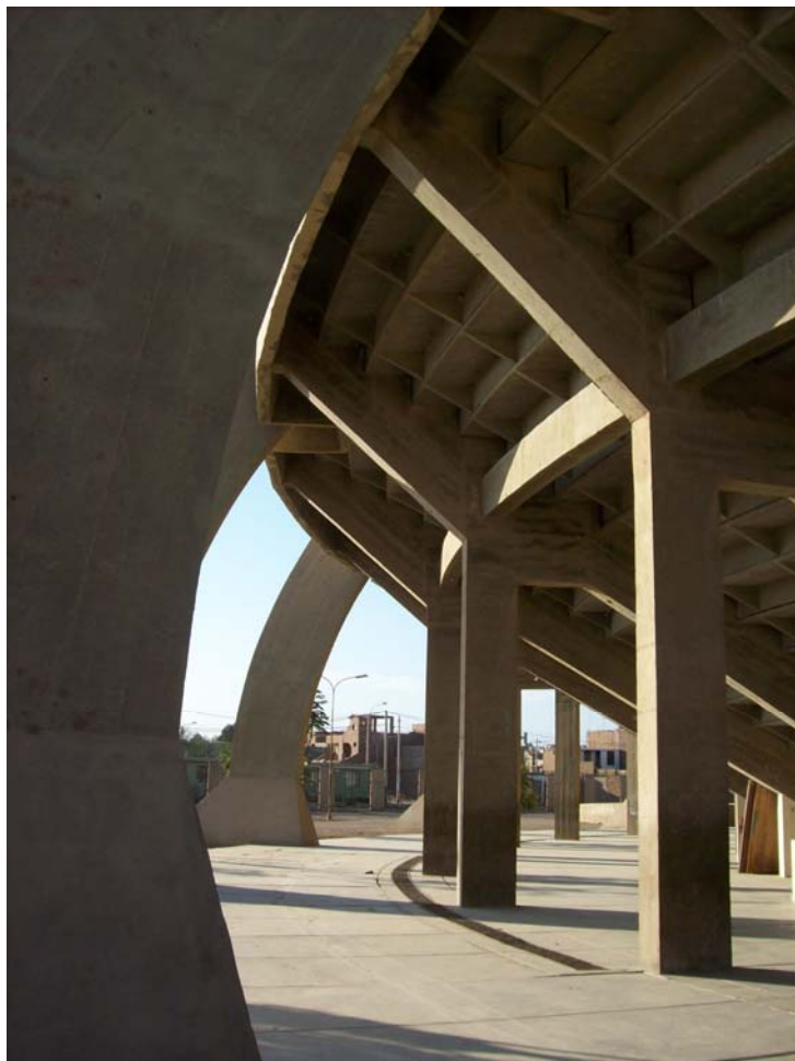
Figure 87. University stadium Ica - no significant damage
