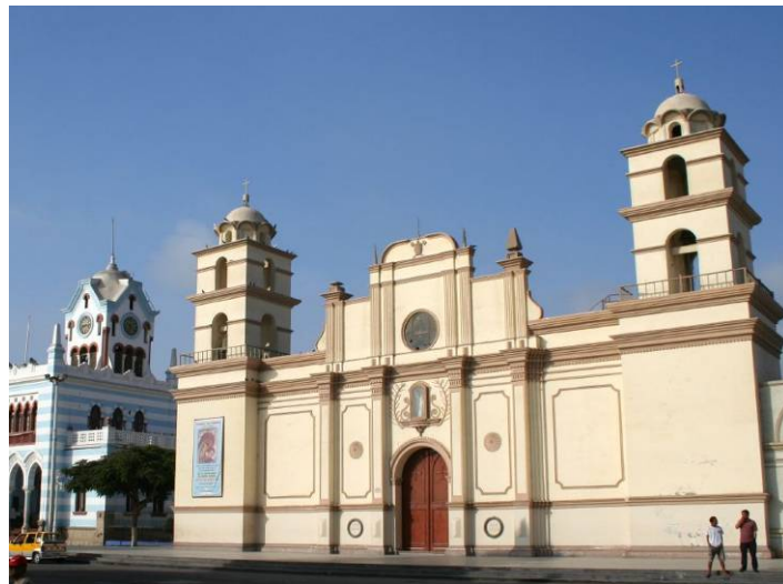
Figure 59. Cathedral San Clemente before Earthquake
