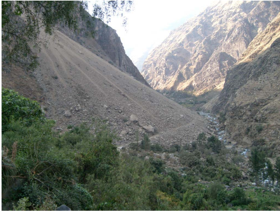
Figure 20. Reactivation of scree slope Photo – Ministry of Transport and Communications
