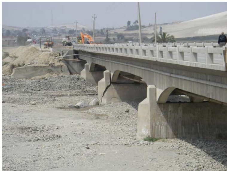
Figure 104. Huamani Bridge on the Pan American Highway at San Clemente
