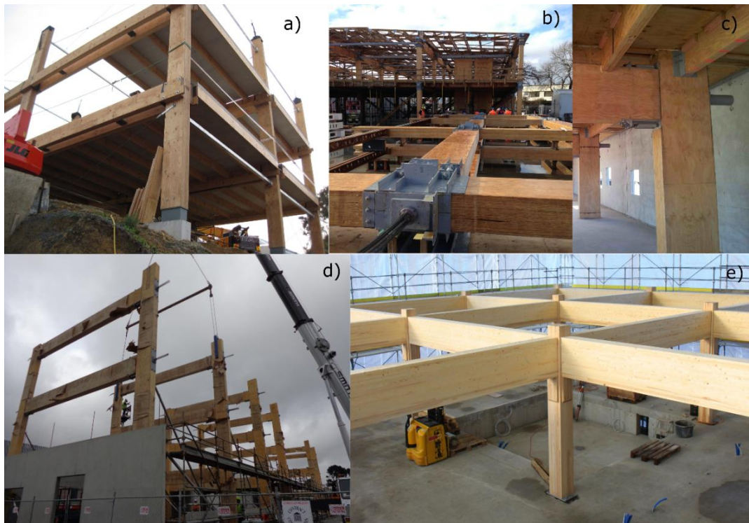
Figure 1: Operative post-tensioned timber buildings: a) Massey University, Wellington (courtesy of Andy Buchanan); b) Trimble Office, Christchurch (courtesy of Paul Drummond); c),d) Merritt Building, Christchurch (courtesy of Andy Buchanan); e) ETH House of Natural Resources, Zurich (Copyright ETH Zurich).
