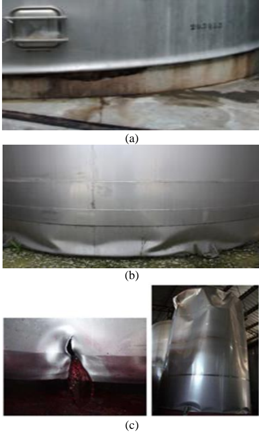
Figure 1: (a) E buckling in 2010 Maule earthquake [5]; (b) D buckling; (c) secondary buckling in 2012 Emilia earthquake [6].
