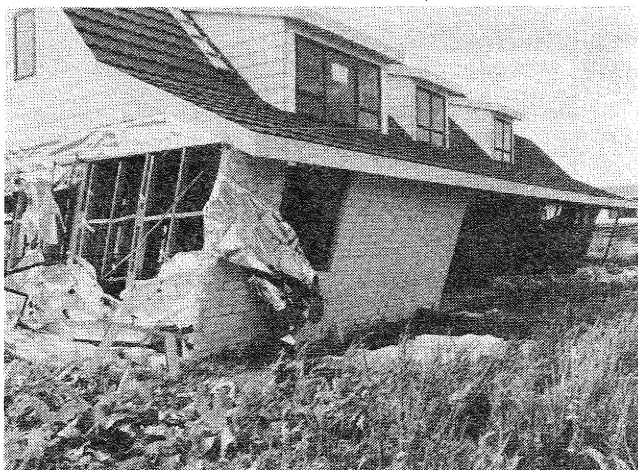
Figure 4.1.10 : House under construction
