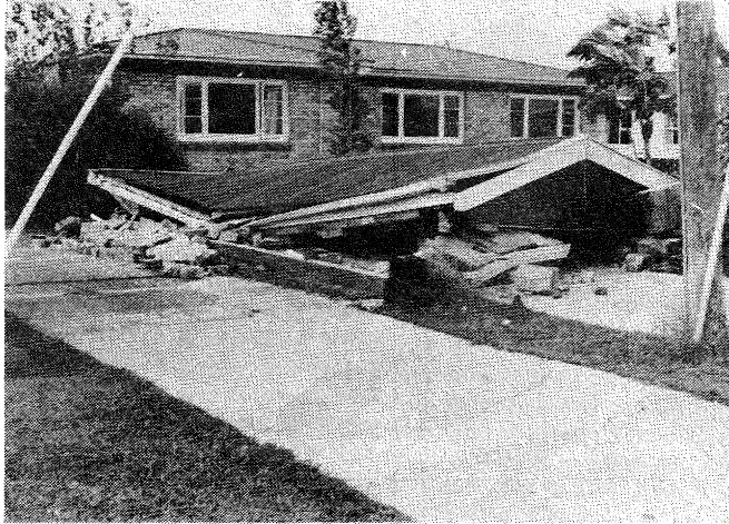
Fig. 4.2.4 : Unreinforced masonry garage
