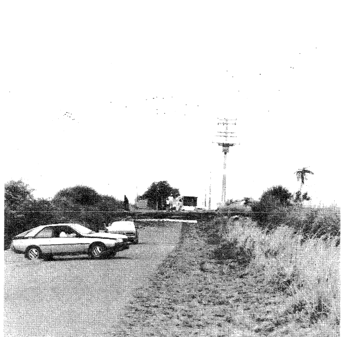
Fig. 3.15 : Damage to McCracken Rd. where it intersects the main fault trace
