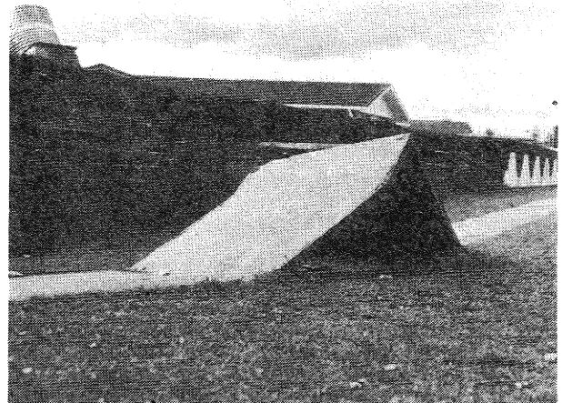
Fig. 2.10 : Compression of the footpath in Edgcumbe
