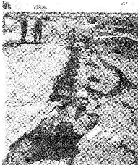
Fig. 3.6 : Cracks in the approaches to the Landing Rd. bridge over the Whakatane River.
