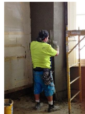
e) application of FRCM in a URM building in Auckland
