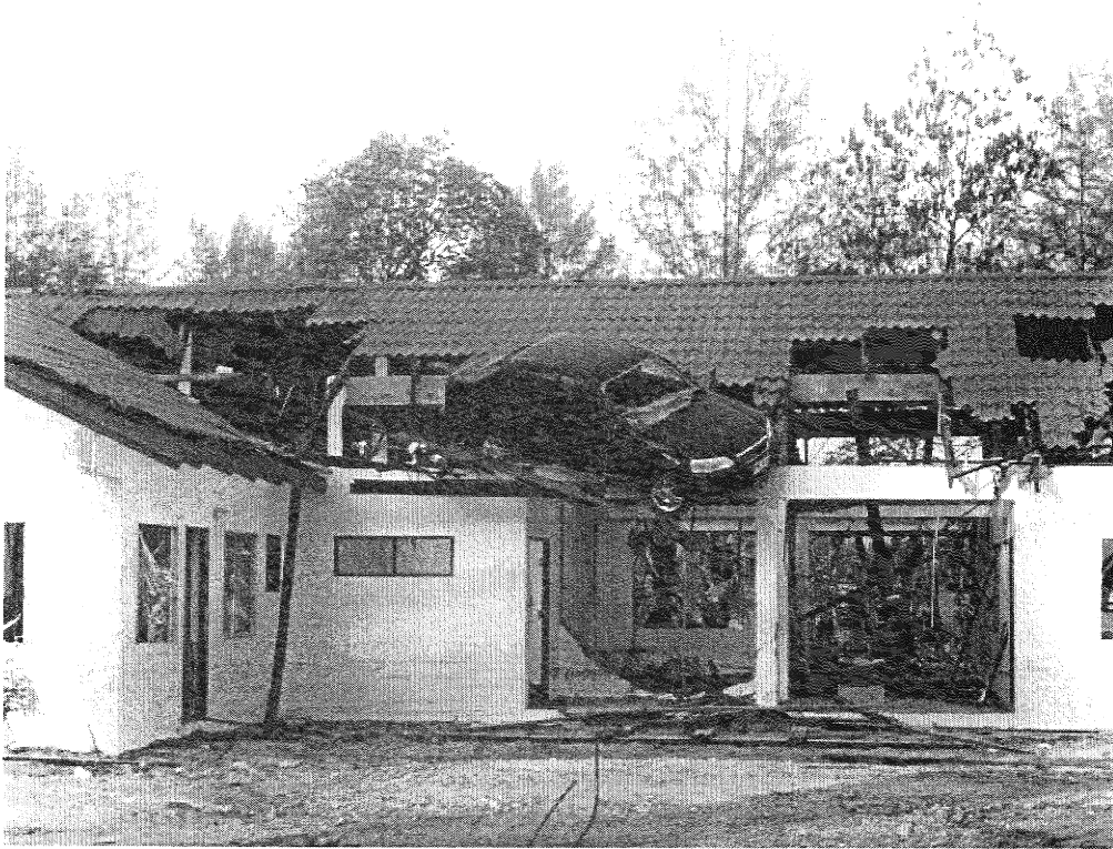
Figure 4. Tsunami wave heights were inferred from strand-lines and watermarks on buildings. In this case a car was lifted above the roofline of a resort in Khao Lak (Photo Thai Meteorological Department).
