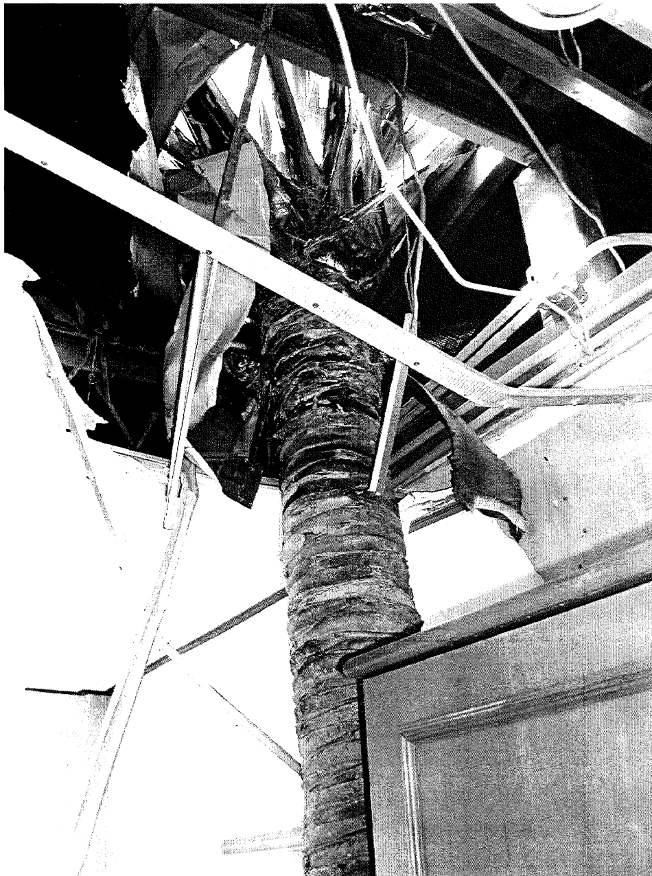
Figure 14. Extraordinary volumes of debris were entrained by the tsunami and contributed to its destructive impact. This coconut palm trunk penetrated the roof and internal ceiling of a hotel on Koh Phi Phi (Photo ED).
