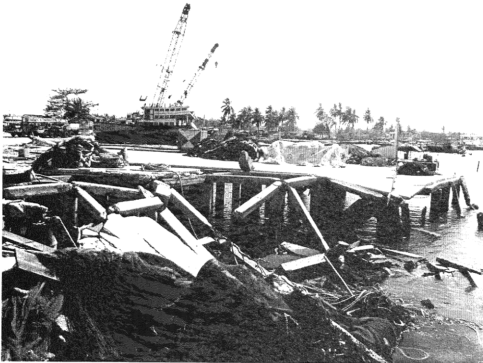
Figure 17. Severe damage to the wharf piles and topping at Ban Nam Kem, a fishing port north of Khao Lak, where the tsunami height reached nine metres (Photo HC).
