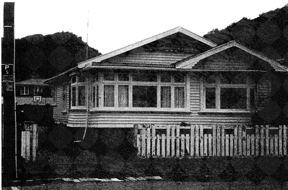
Figure 2. The most common type of pre-1968 West Coast house, one-storey with a corrugated iron roof, weatherboard cladding and (unbraced) pile foundations.
